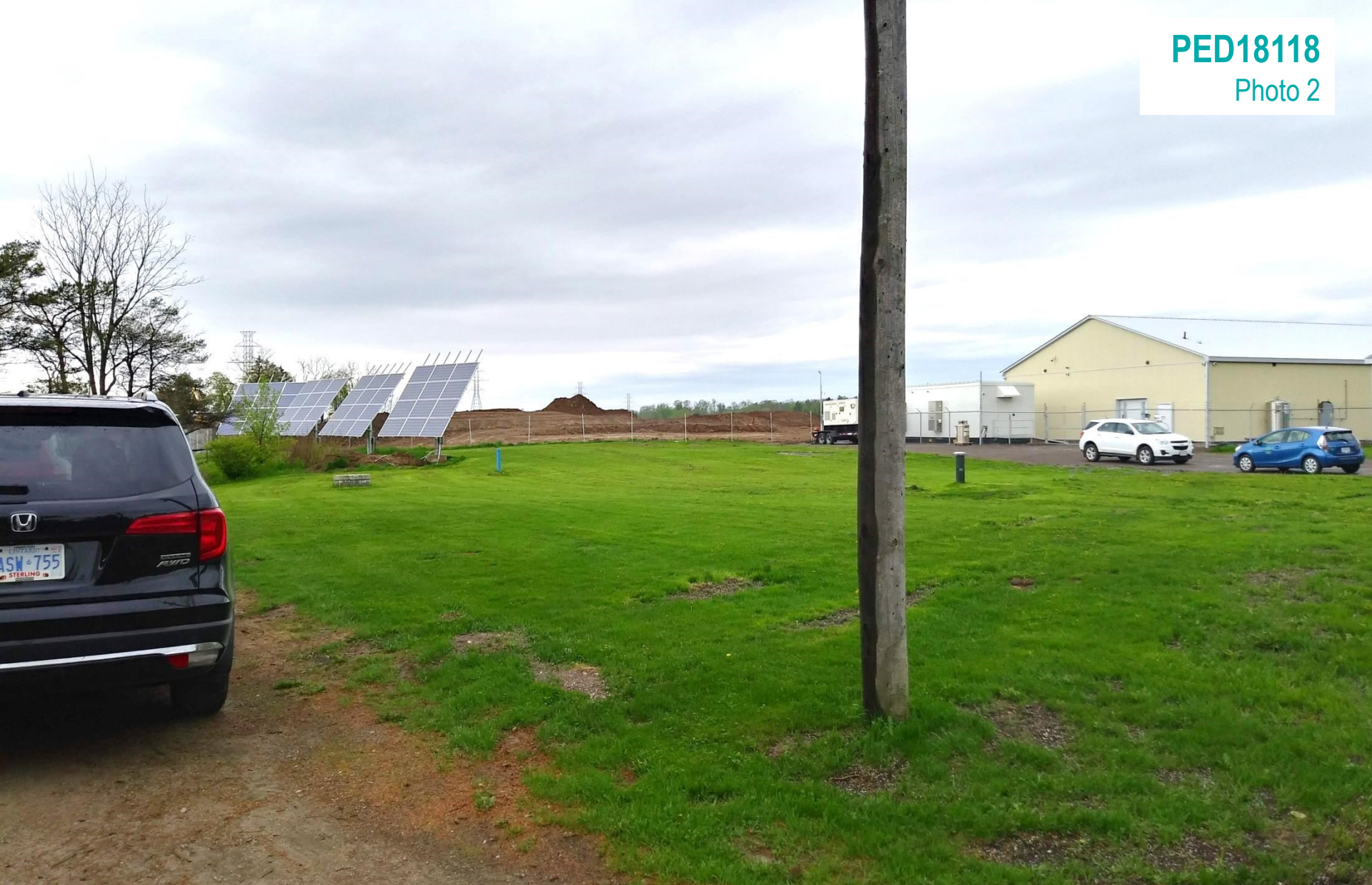
Existing medical marihuana facility and site preparation for DA-17-082
