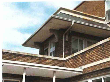
Sundeck (original brackets and roof flashings)
