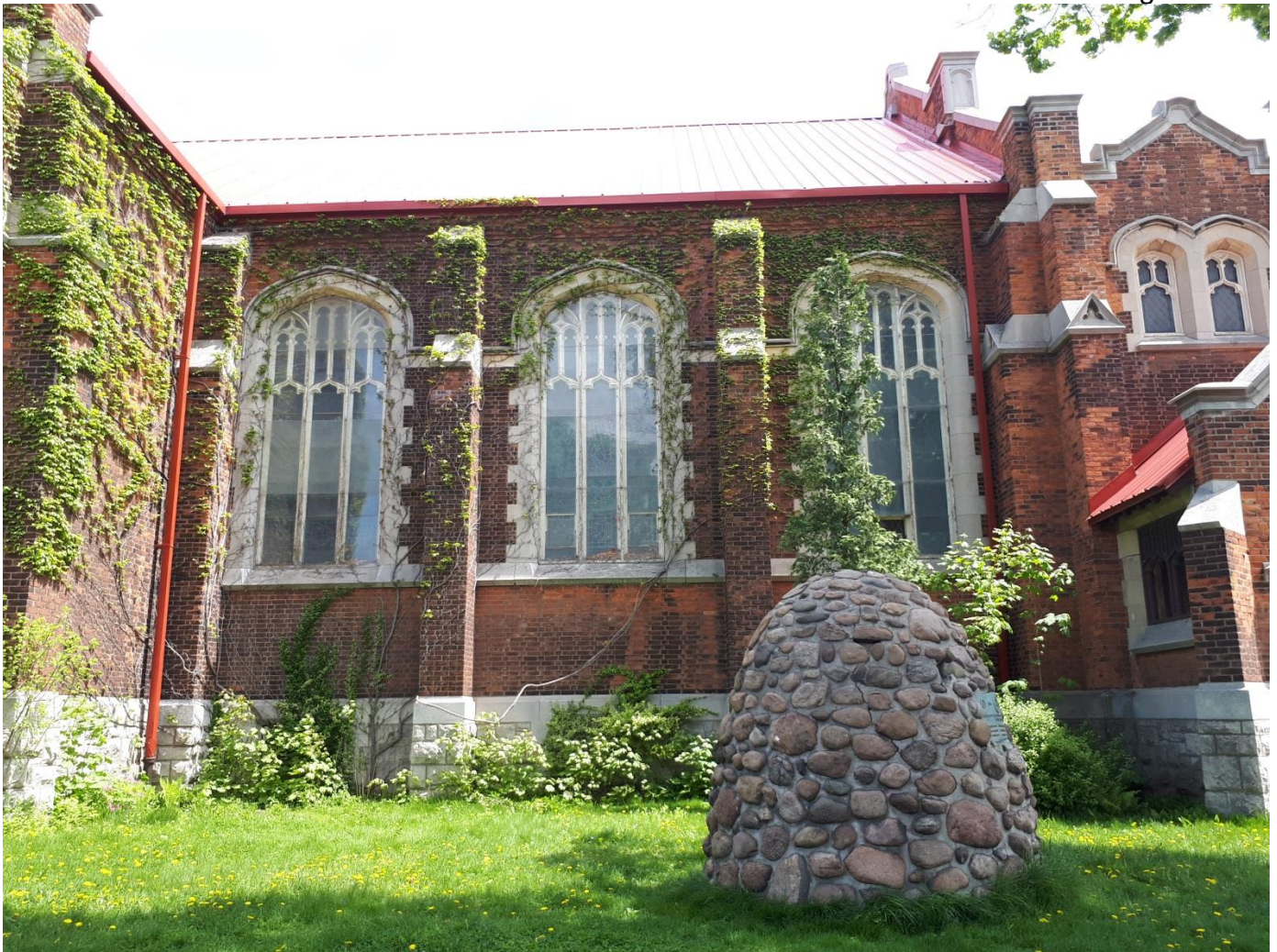
West Elevation Gothic arched window and WW1 cairn, May 18, 2018
