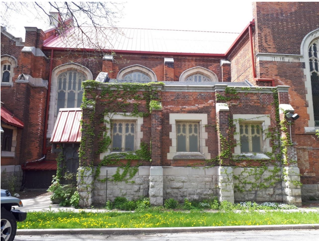
Close up of East elevation addition, May 18, 2018
