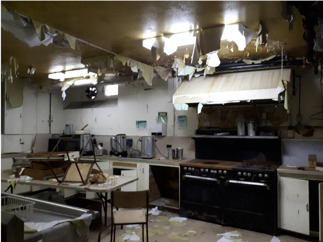
Basement kitchen, May 31, 2018
