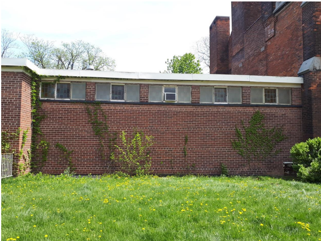
Close up of 1958 addition, May 18, 2018
