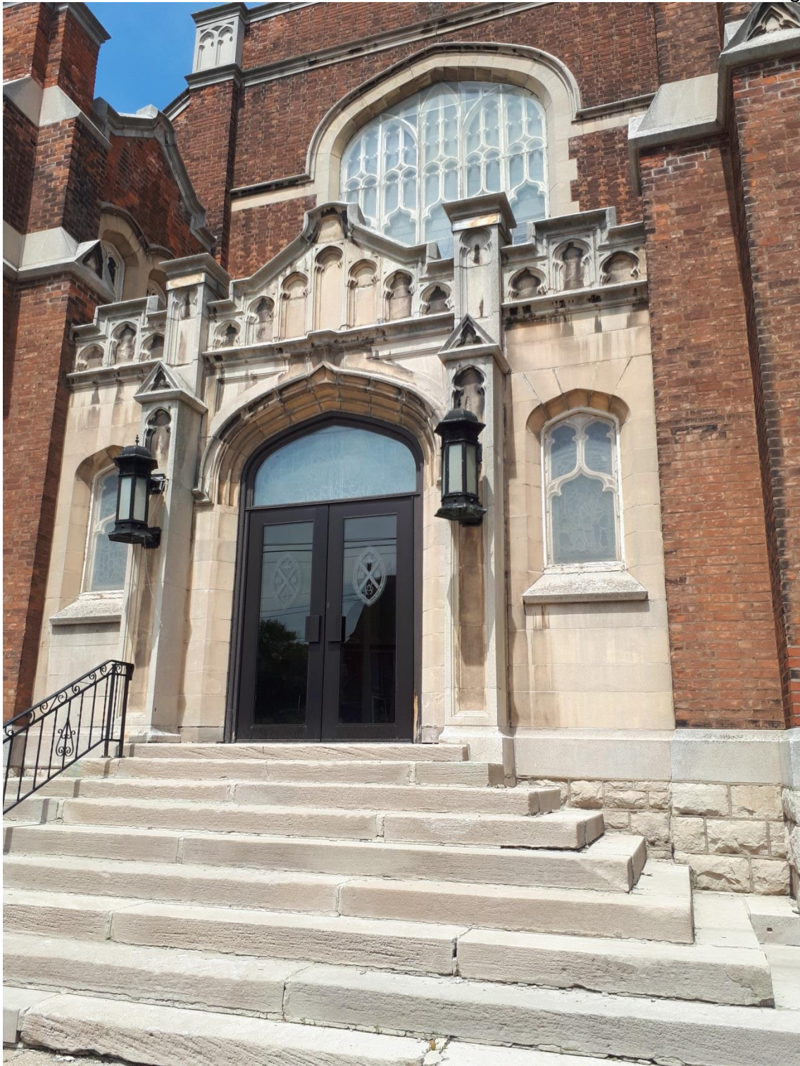
Front Entrance Close-up, May 18, 2018
