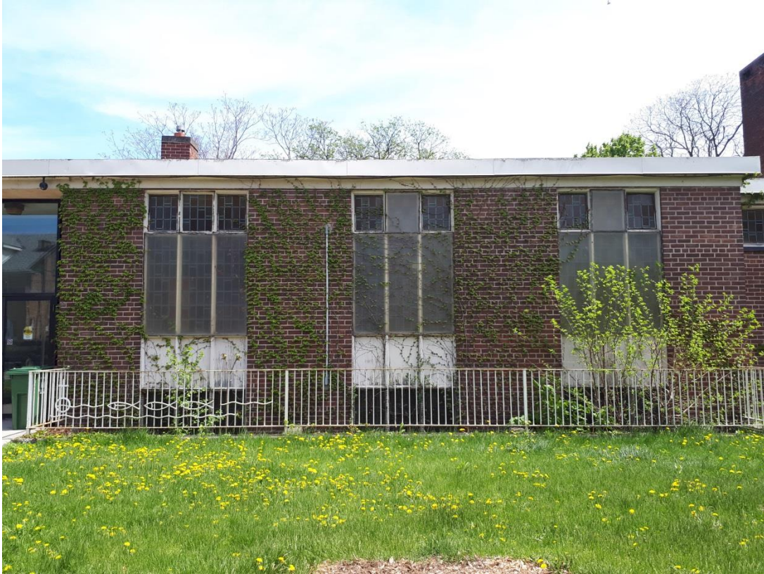
Close up of 1958 addition, May 18, 2018
