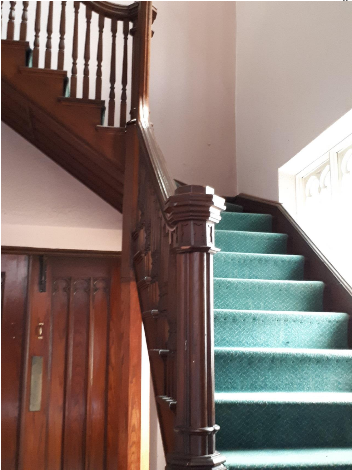
Stairs on east side of front entrance, May 31, 2018
