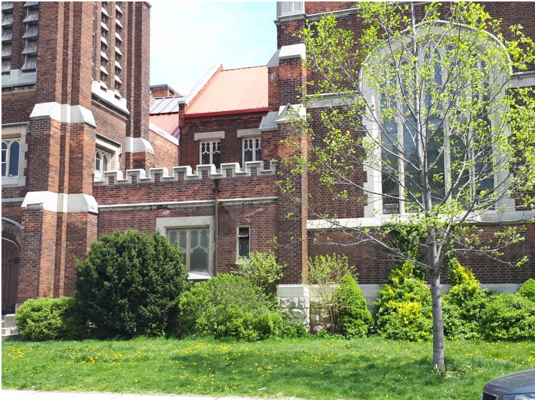
Close up of West Elevation between bell tower and transept
