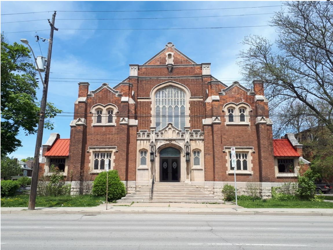
Front Façade, May 18, 2018
