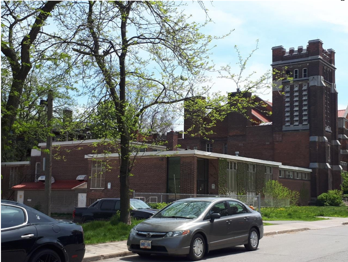
North Elevation including 1958 addition, May 18, 2018
