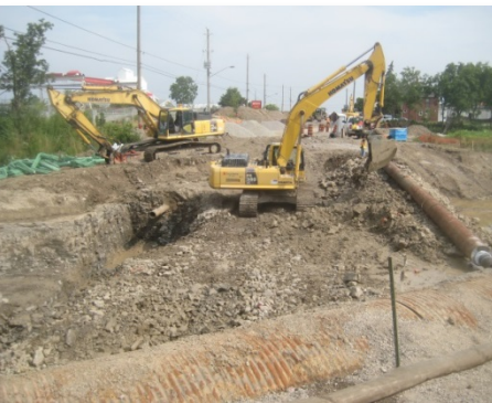
Dartnall Road Culvert
