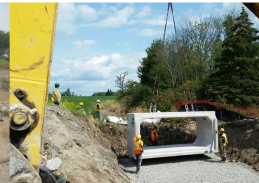
Bell Road Culvert Replacement
