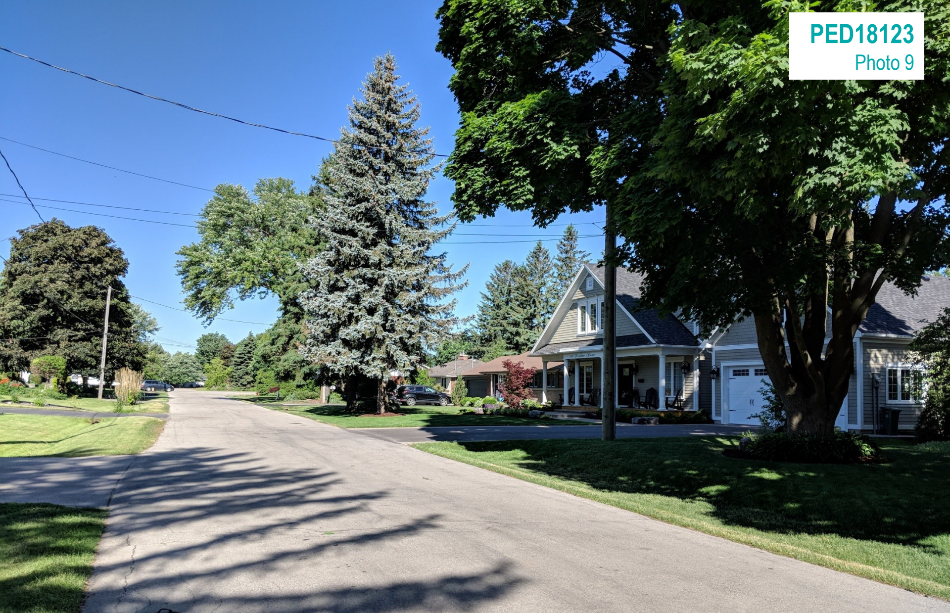
Example of housing stock on Roselawn Avenue
