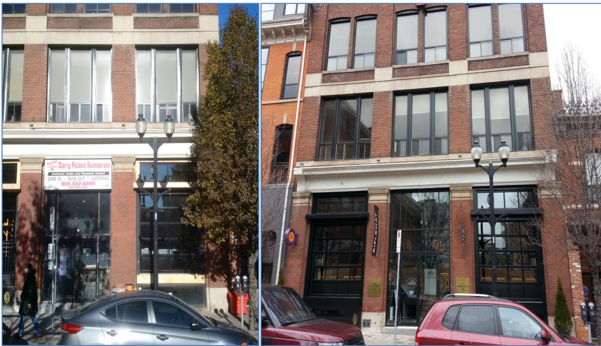
43 King William Street, Hamilton (before and after)
