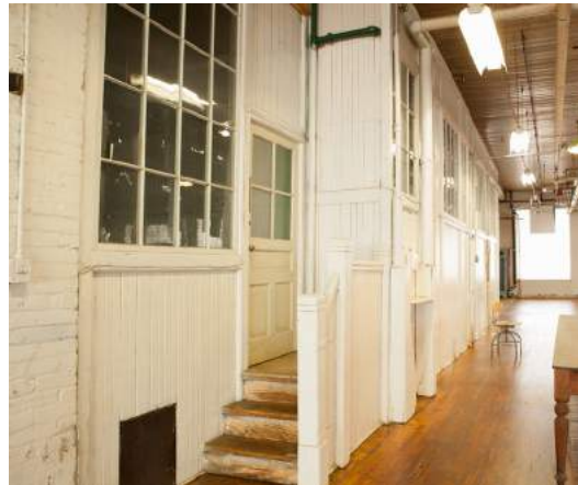
Figure 4.19 - Level 3: An interior wall that seems to be characteristic of an exterior envelope. It has similar character defining windows to those of the exterior and shows a progression of construction.
