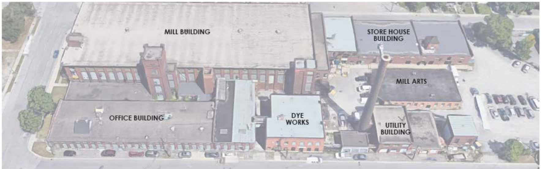
Figure 6.1 - (source: Google Maps) 270 Sherman Complex South View
