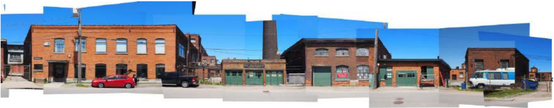
South Elevation of Complex. Source: Heritage Cultural Assessment by mcCallum Sather Architects
