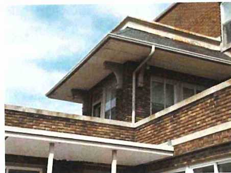
Sundeck (original brackets and roof flashings)
