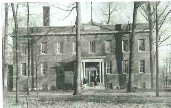
Early Photo - Long & Bisby Building
