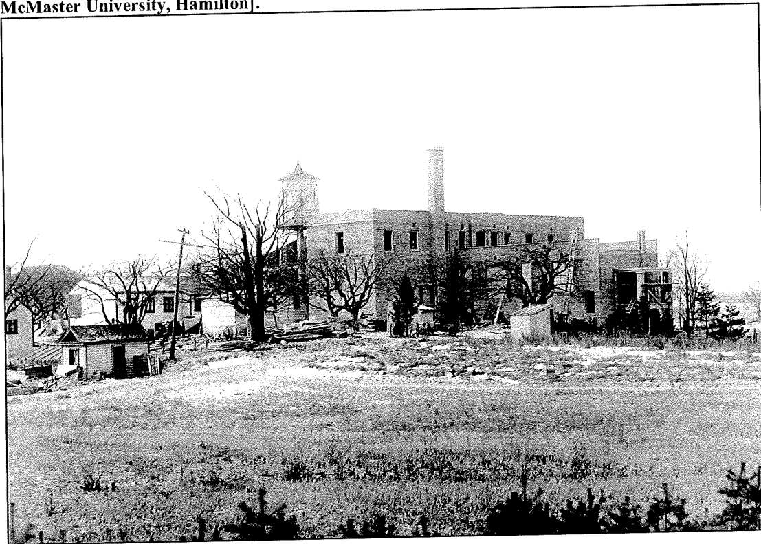
Bruce Building, northeast corner during construction. Circa 1920. [Health Sciences Library, McMaster University, Hamilton].
