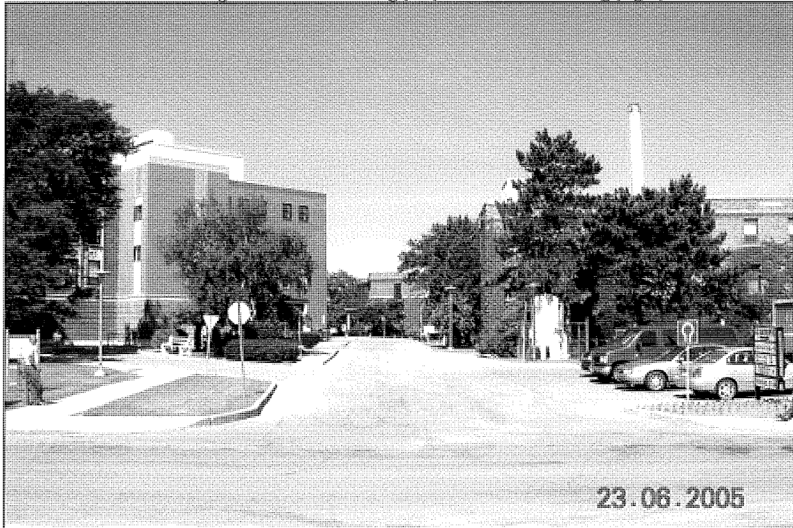
View west to Bruce Building with Wilcox Building (left) and Central Building (right).
