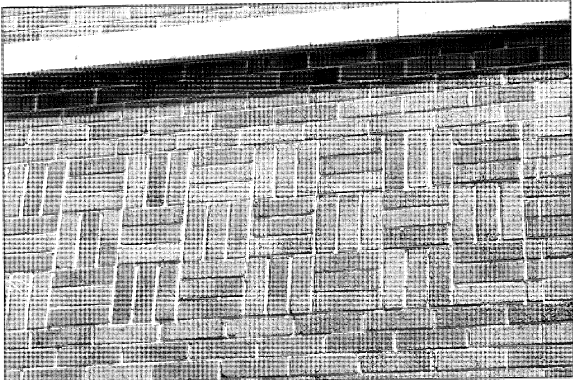
Detail of the checkerboard brickwork located on the southeast wall.
