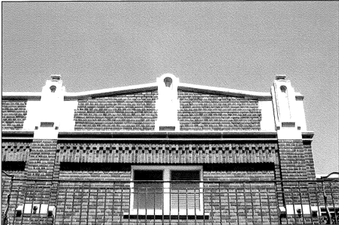
A pedimented parapet with concrete detailing highlights the end bays of the southwest wall.
