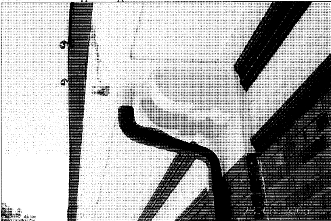
Paired wood brackets support the upper verandah.
