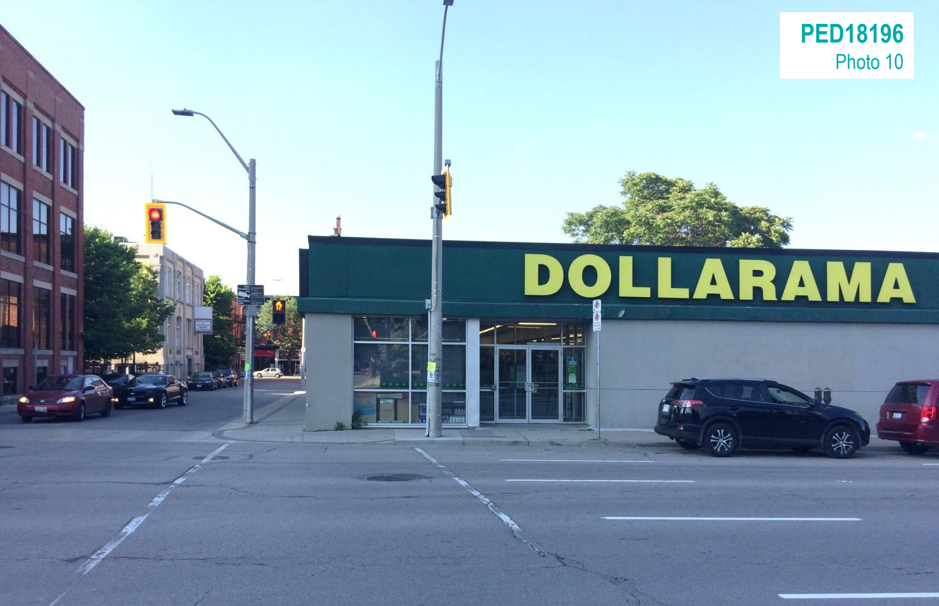
Existing development at 157 Main Street East located to the north of the Subject property, as seen from Main Street East looking north
