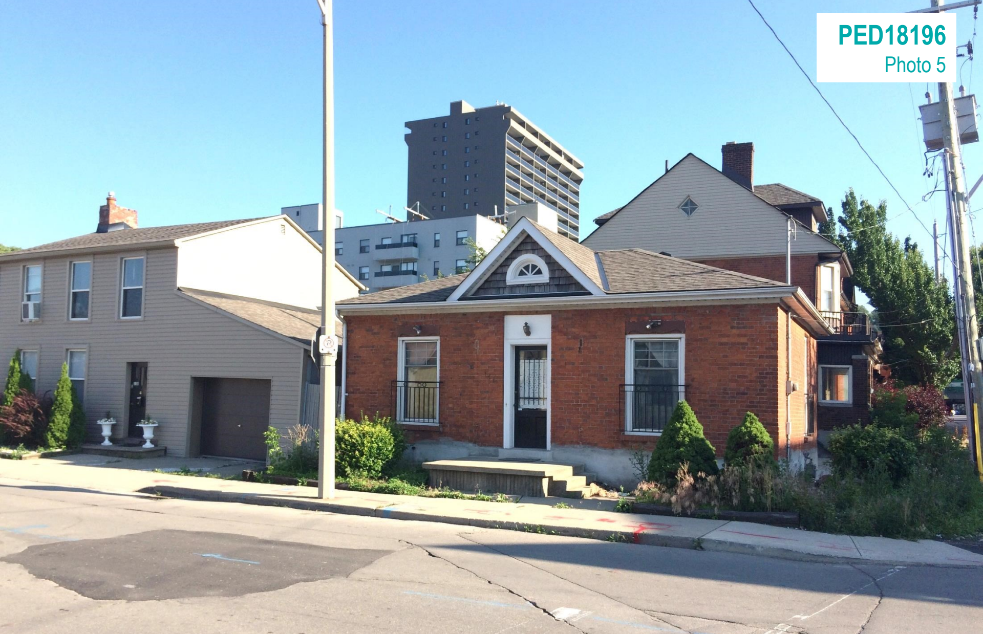
Existing development at 154 and 158 Jackson Street East located to the south of the Subject property, as seen from Jackson Street East looking south west
