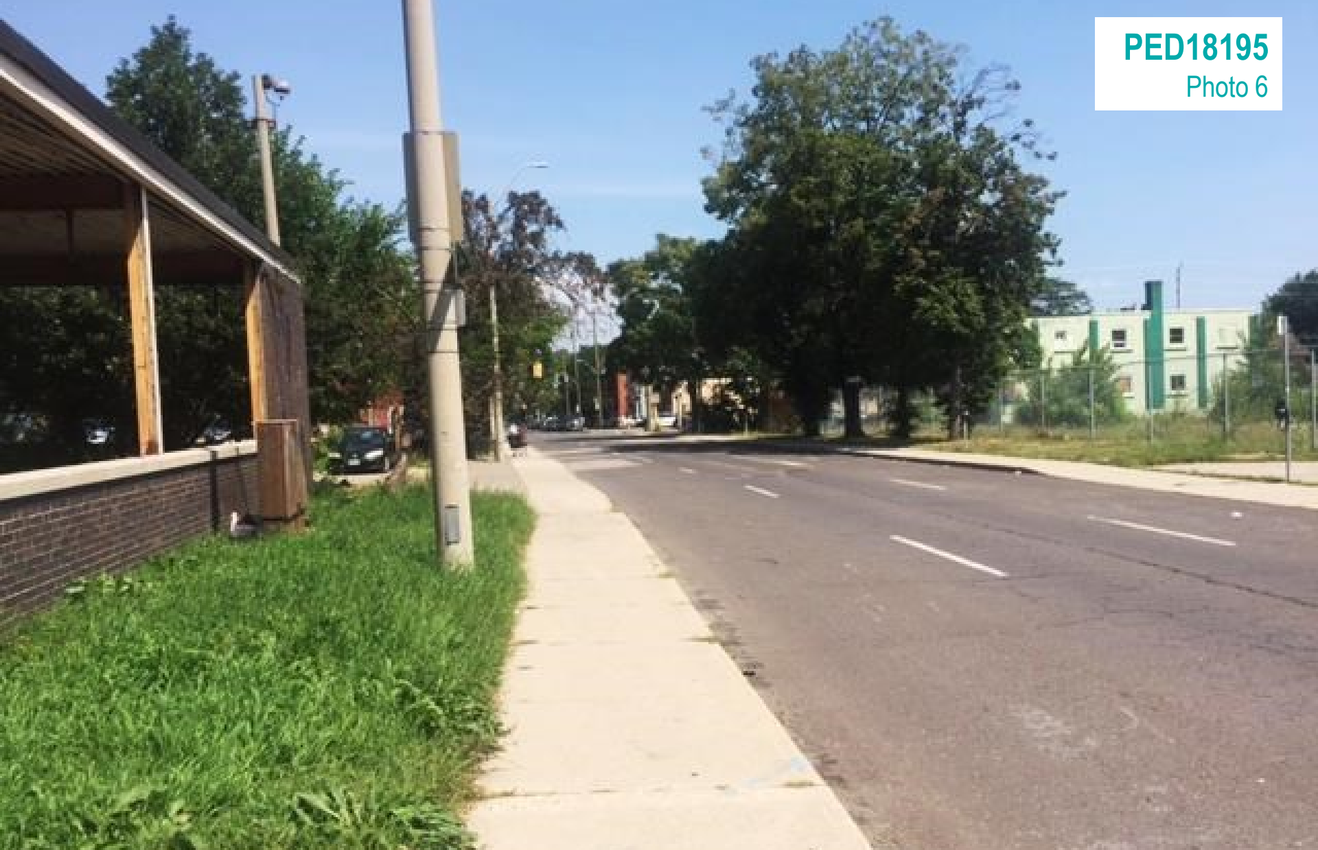
Looking north along Catherine Street North
