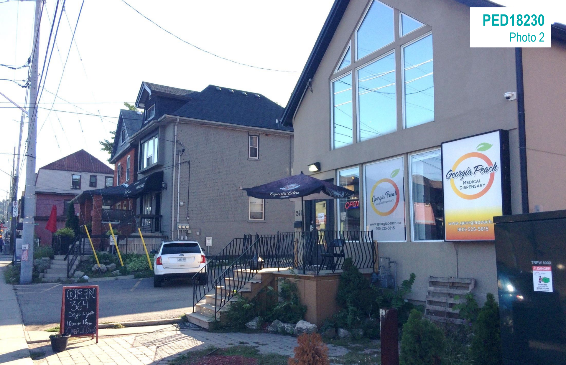
246 Dundurn Street South located to the south of the Subject Property, as seen from Dundurn Street South looking south west
