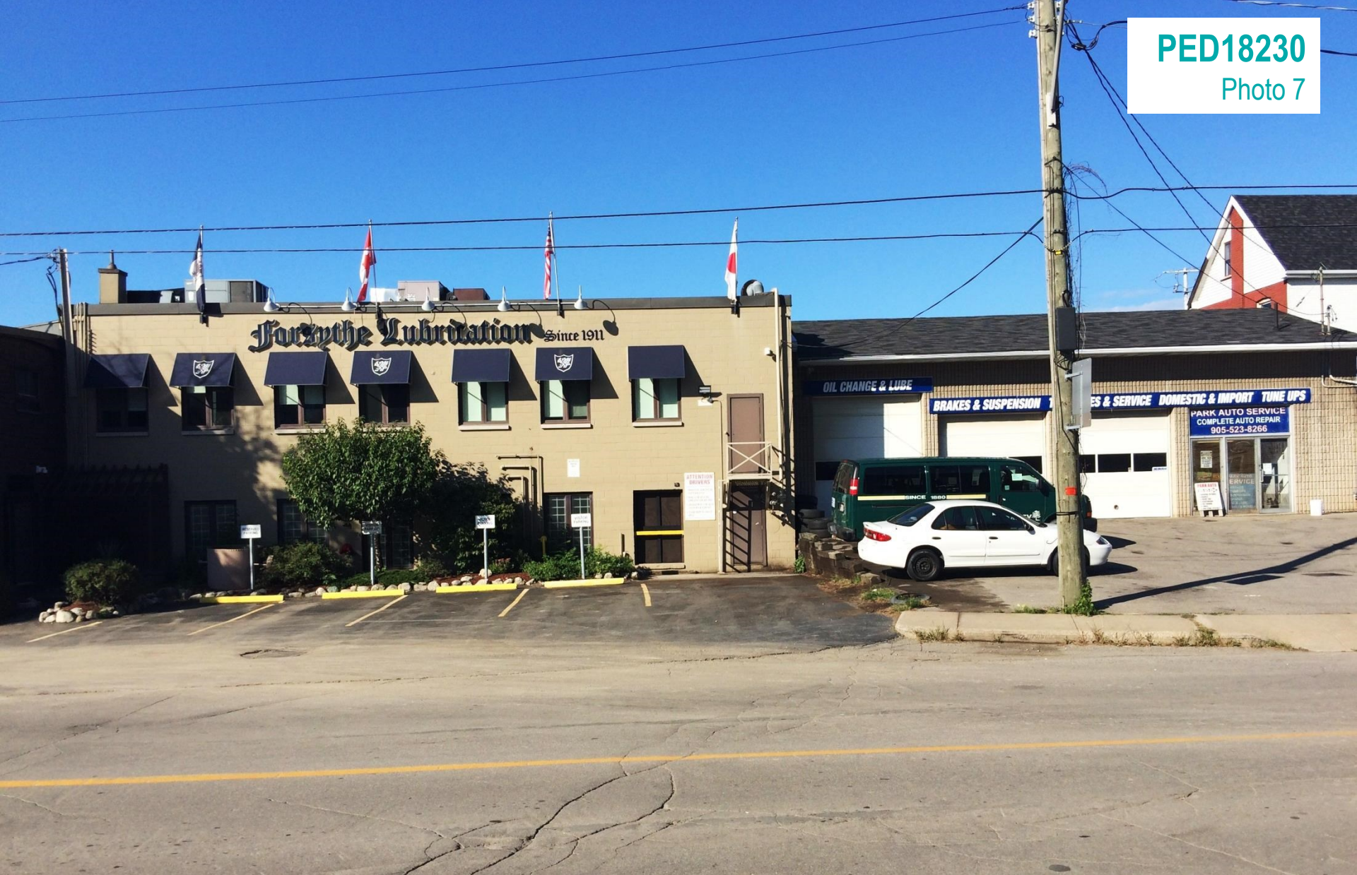
120 Chatham Street located to the north of the Subject Property, as seen from Chatham Street looking north
