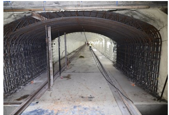
Mountain Trunk Storm Sewer Rehabilitation
