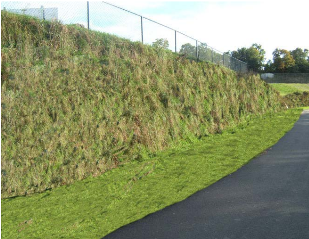
Figure 6.19 Mechanically Stabilized Earth Berm (Strata System)
