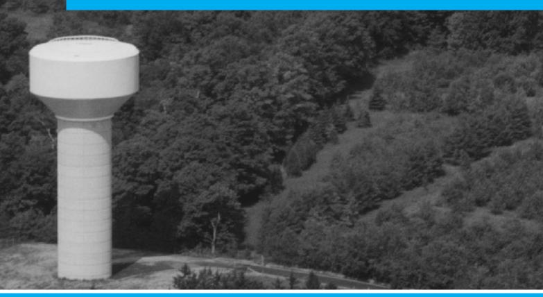
The Freelton water supply system consists of two wells, one elevated water storage tank, treatment, sampling and analysis which services a population of approximately 790 people. The water source for the community of Freelton is ground water.
