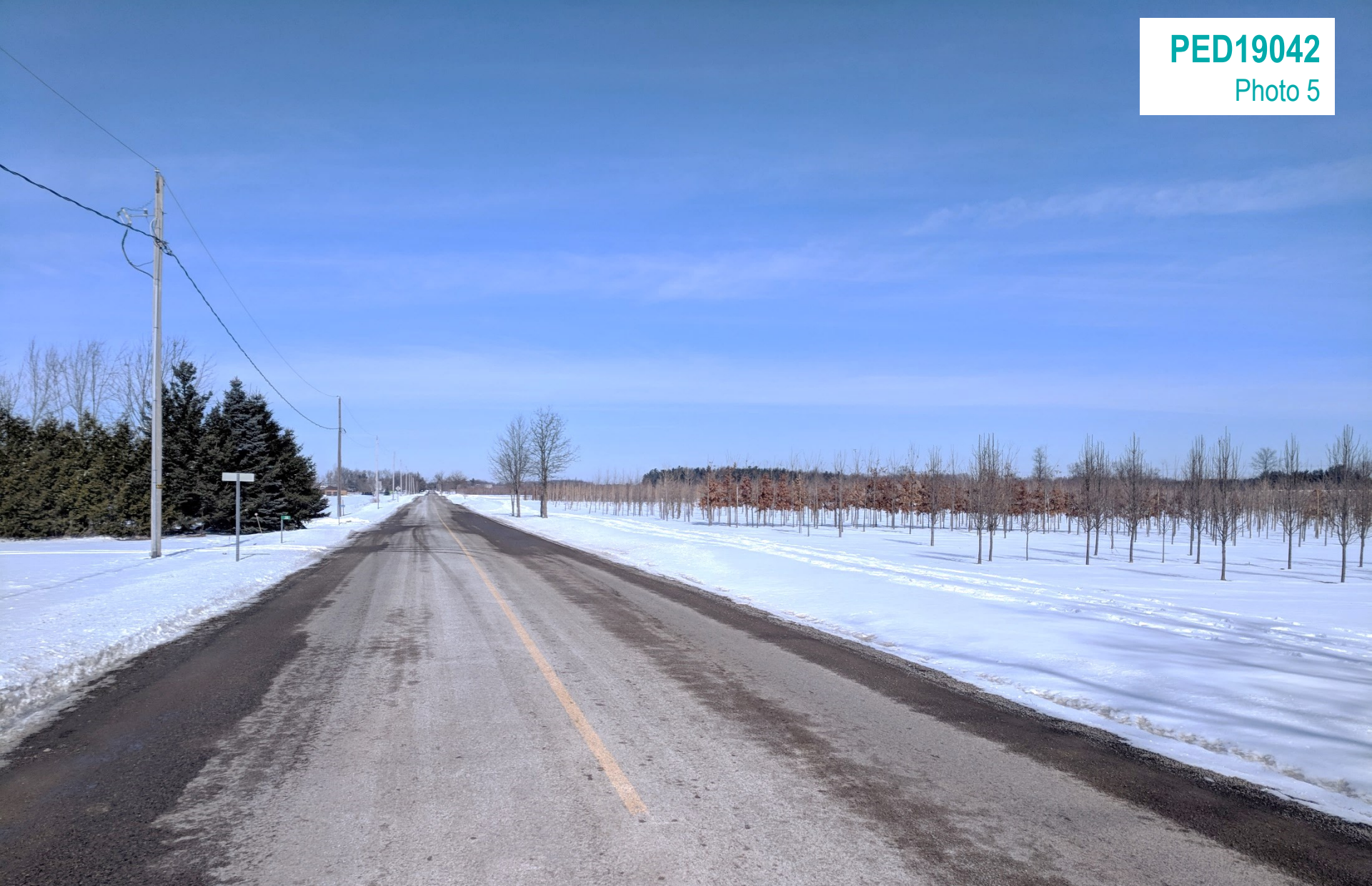
Looking north on Orkney Road at the nursery
