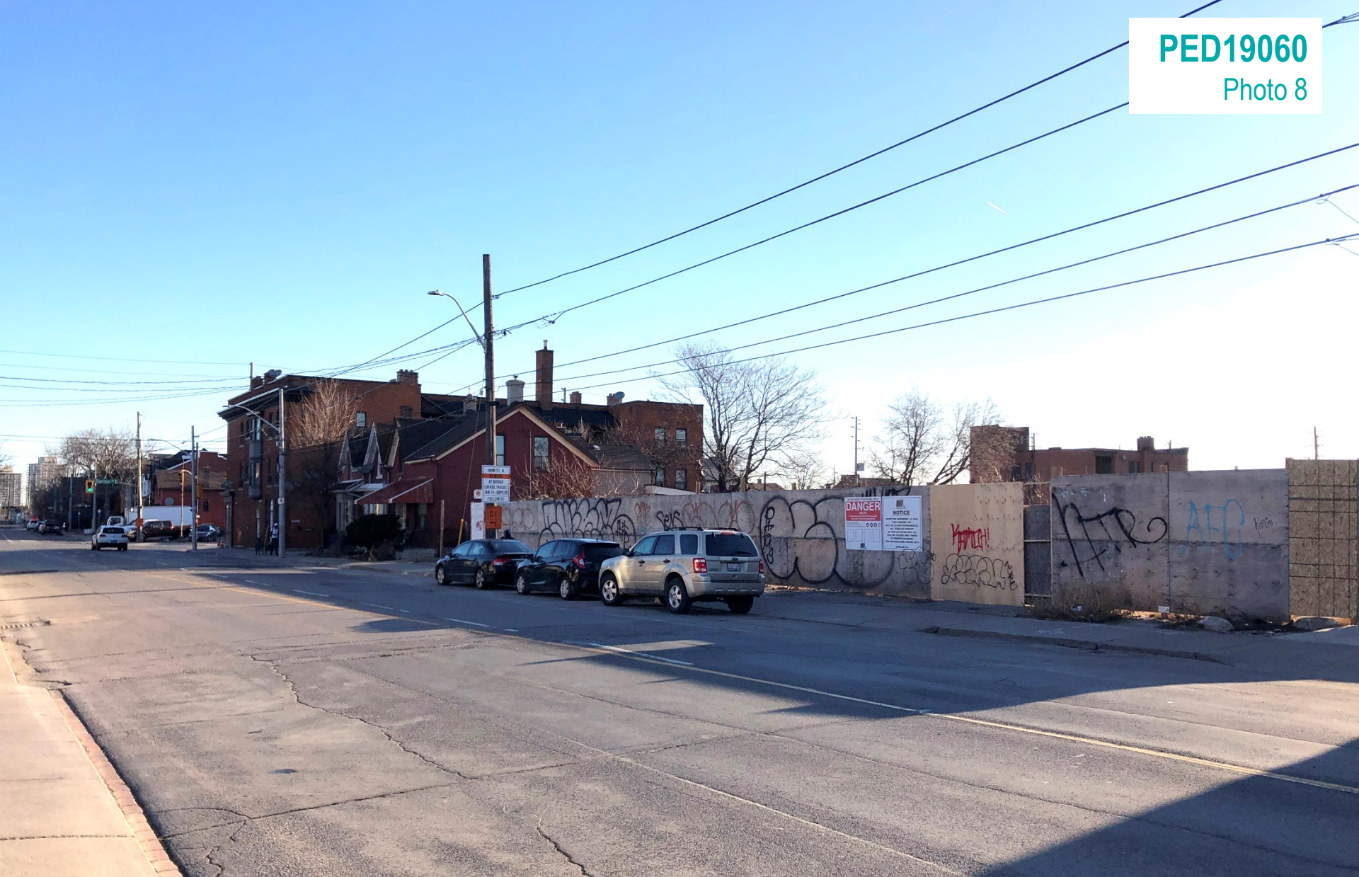
Subject lands looking north on John Street North
