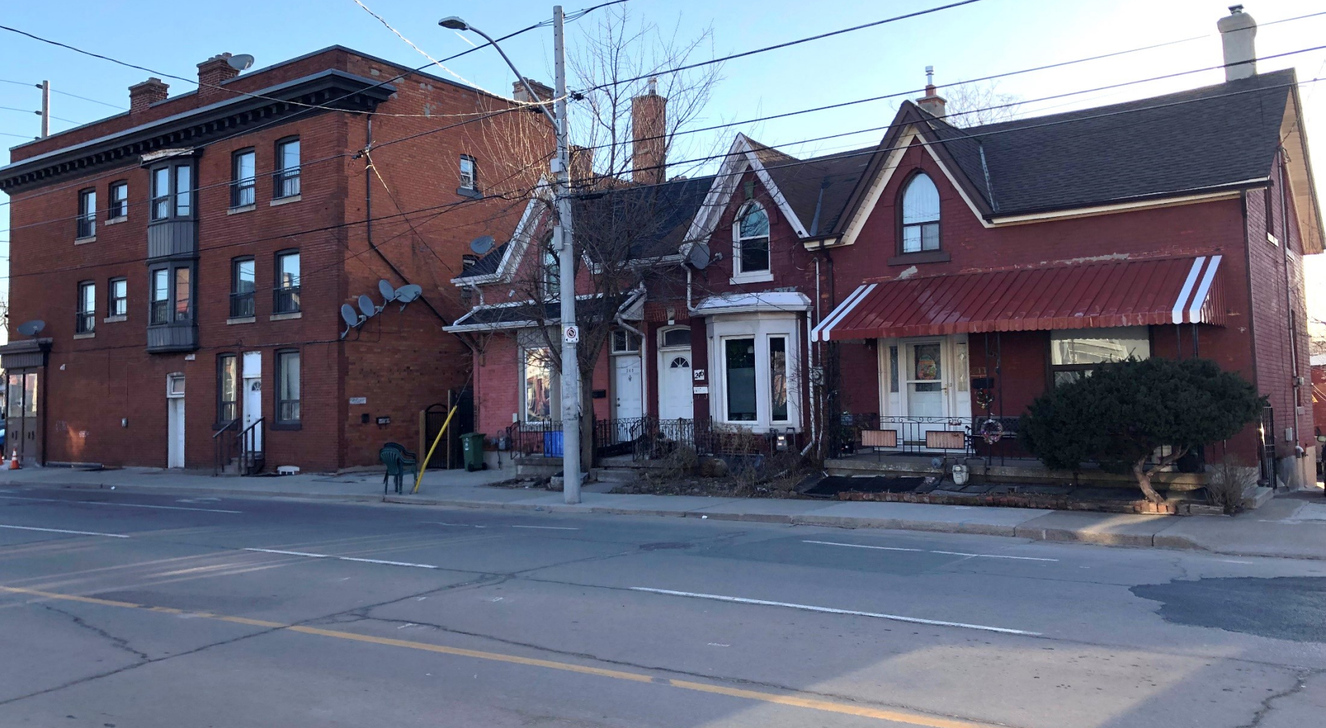
Abutting lands along John Street North
