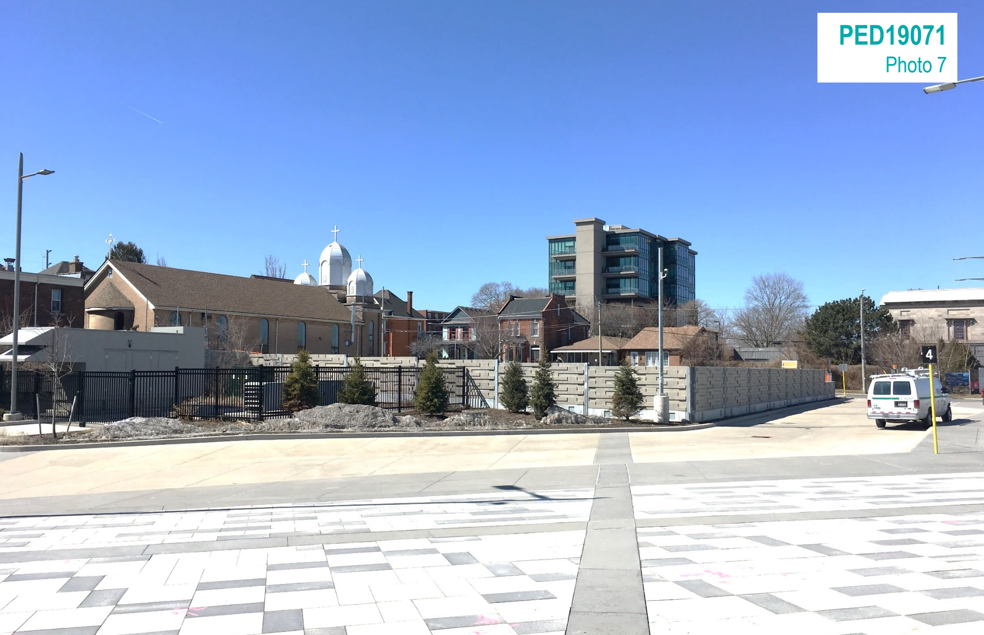
Subject lands, as seen from the GO Bus Station looking southwest
