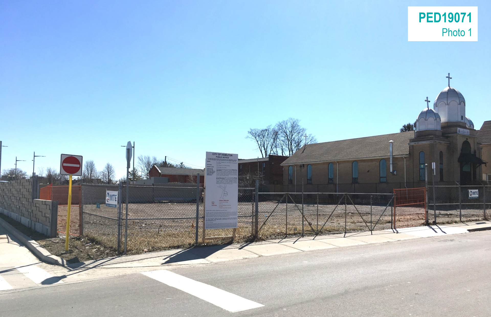
Subject lands, as seen from the intersection of Stuart Street and MacNab Street North looking southeast
