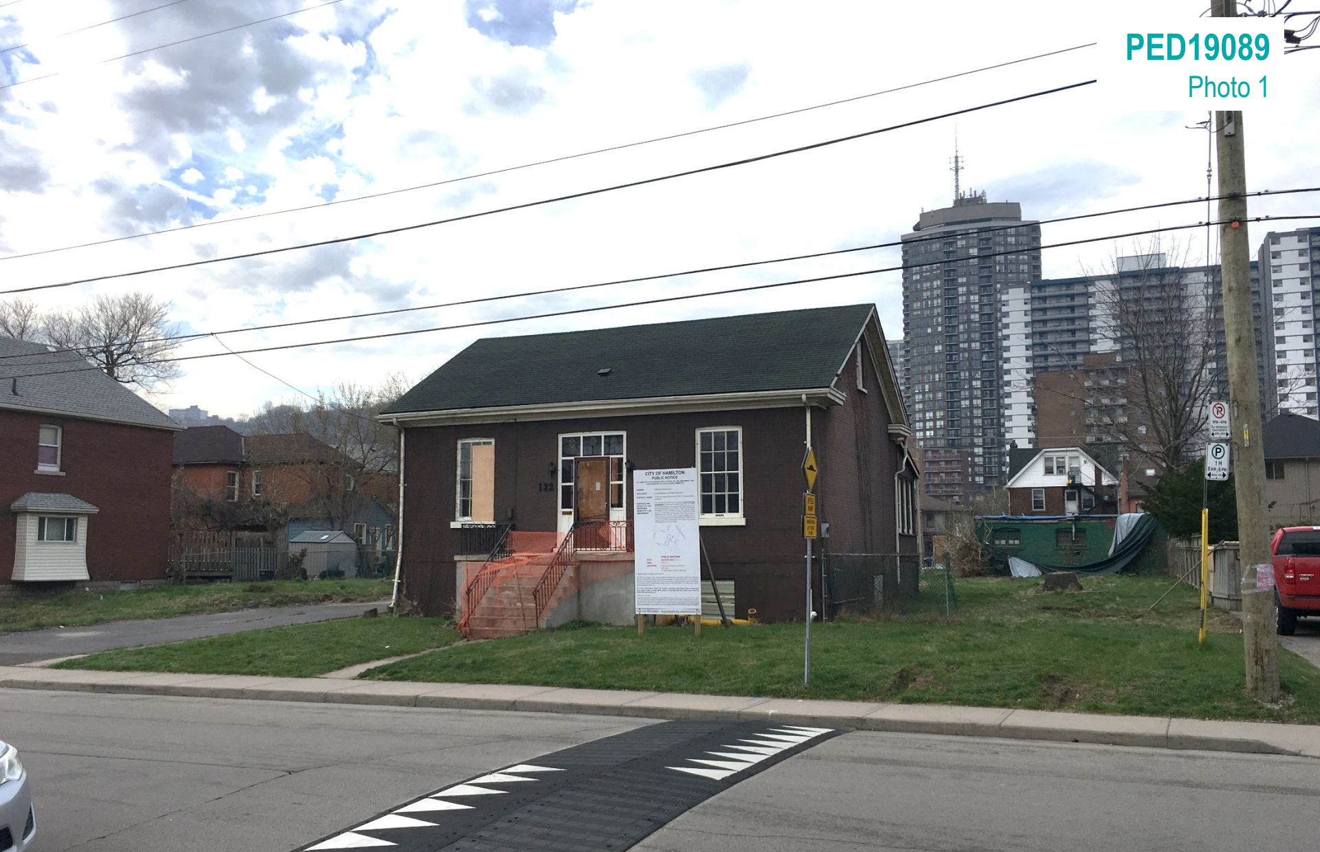
Subject Lands as seen from Augusta Street looking south.
