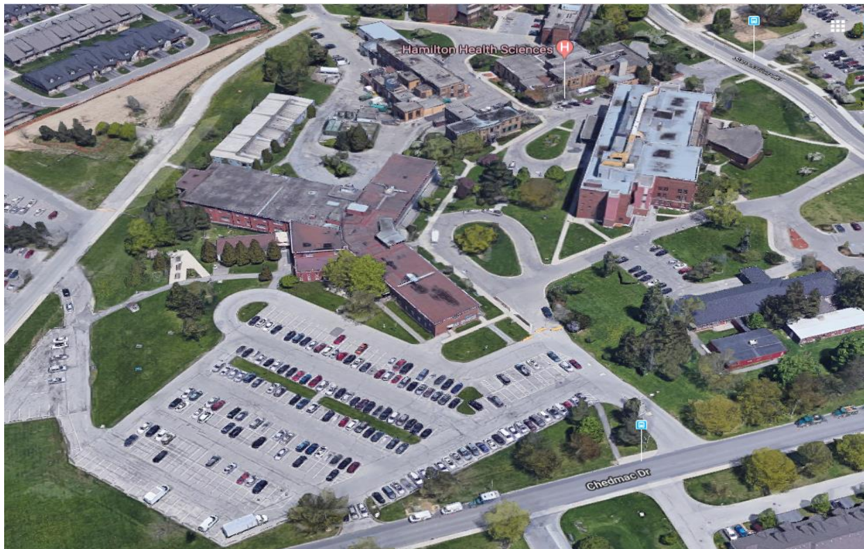
Existing Conditions – 555 Sanatorium Road – 8 Buildings
