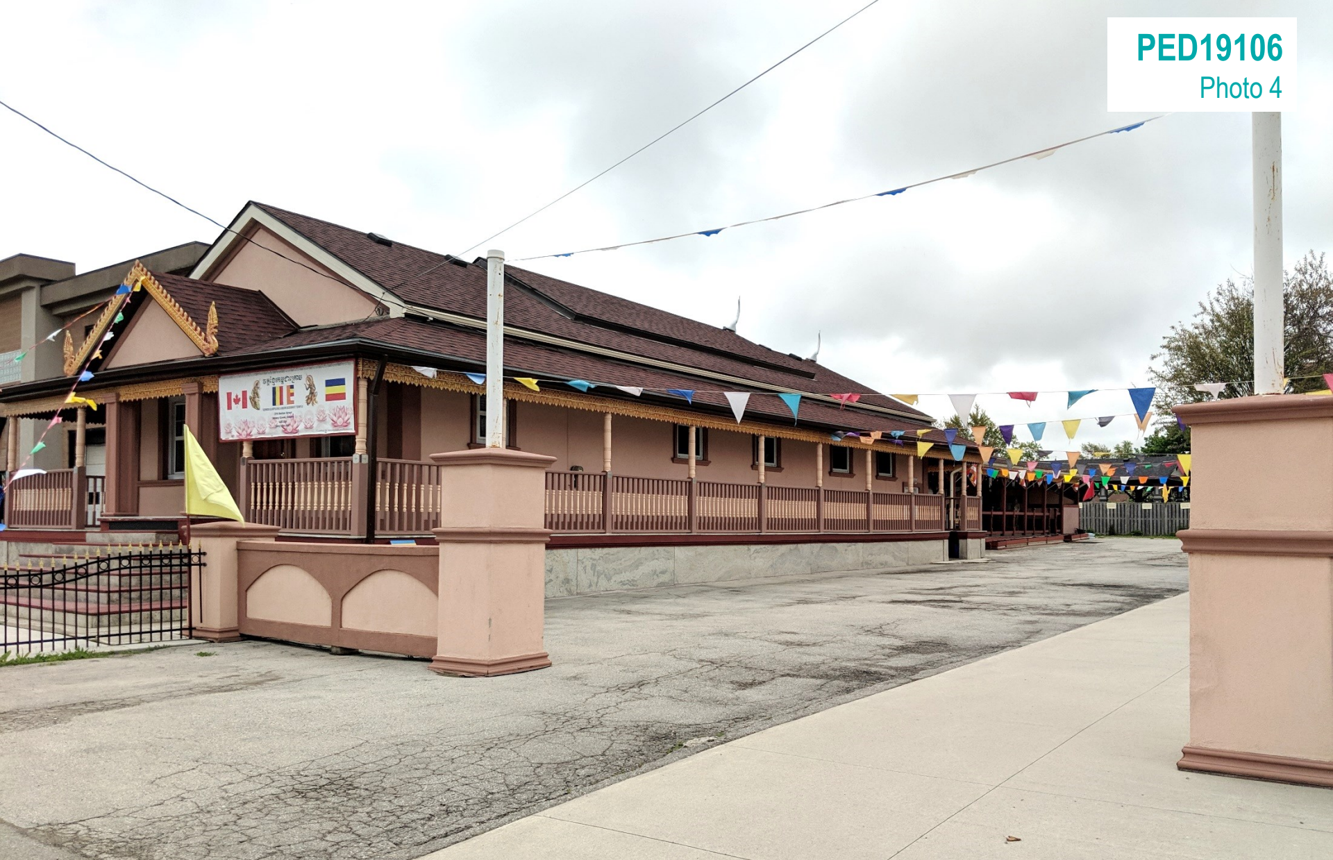
Parking area within Subject Lands.
