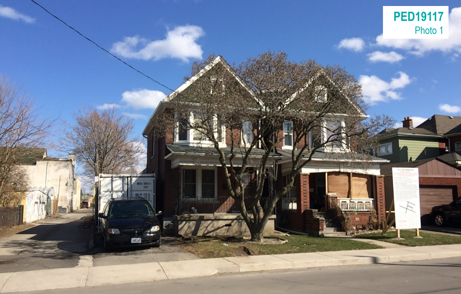
Existing semi-detached dwelling on the subject property, as seen from Barnesdale Avenue North looking east
