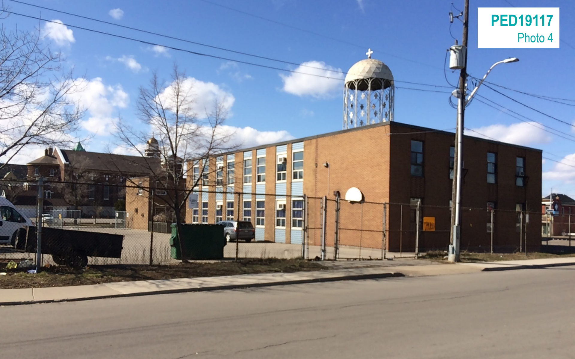
Existing place of worship located at 728 and 732 Barton Street East, located to the west of the subject property, as seen from Barnesdale Avenue North looking north west
