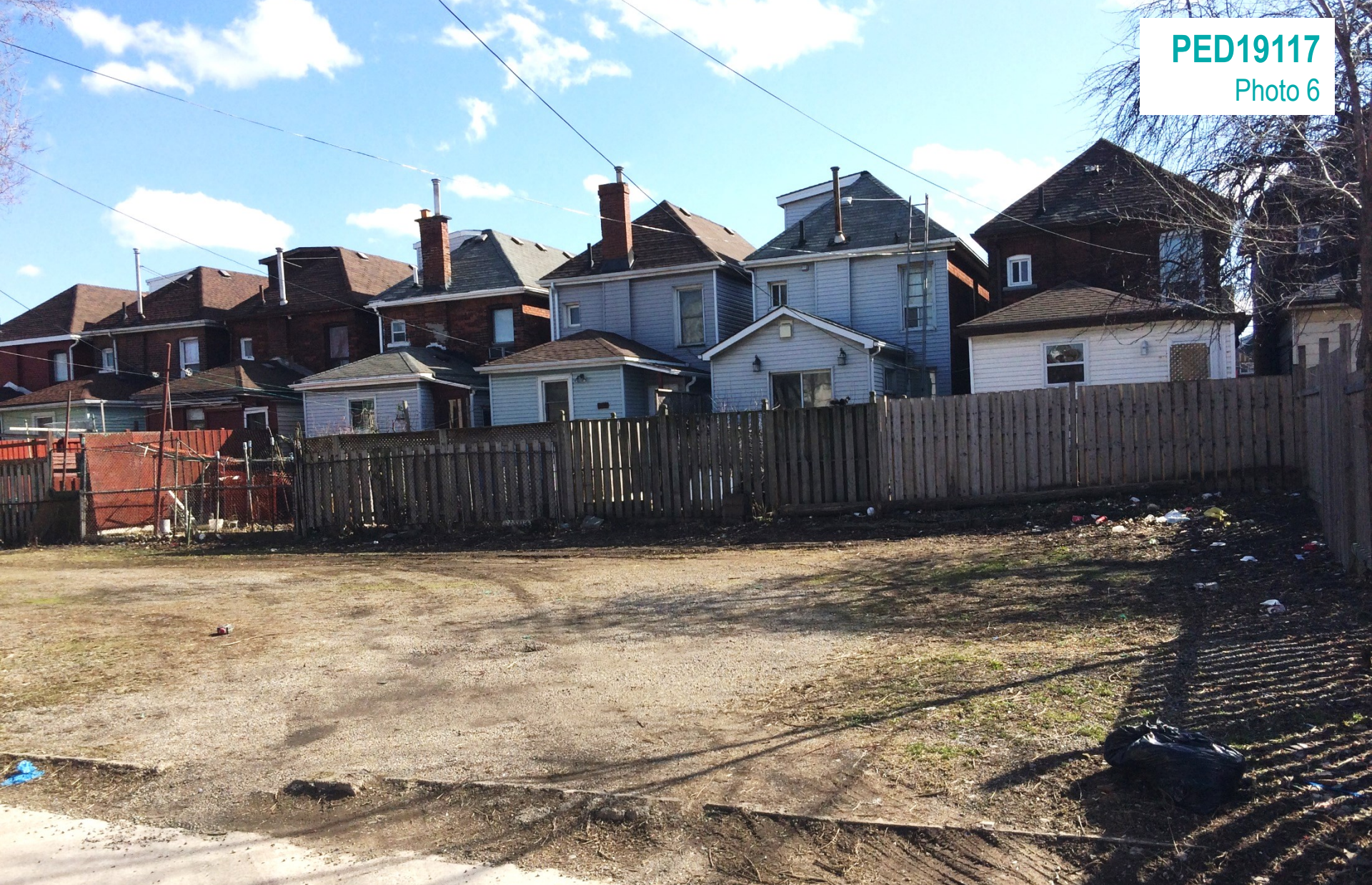
Rear of the subject property, as seen from alleyway looking south east
