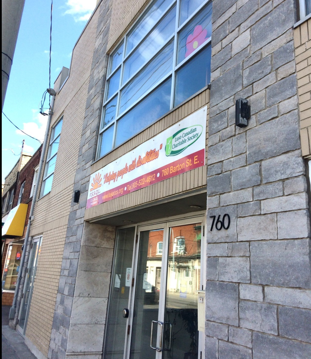
Existing building at 760 Barton Street East, as seen from Barton Street East looking south east
