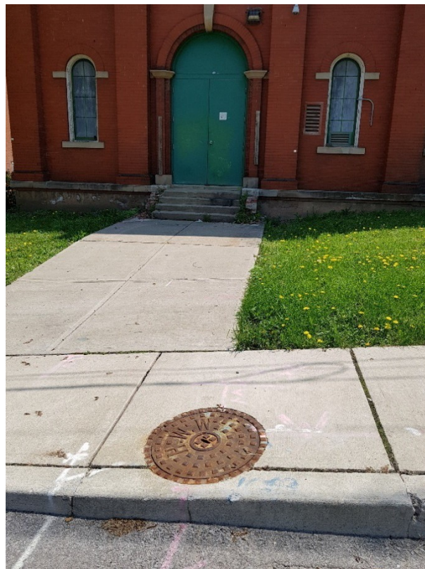
Figure 29: 'HWW' (Hamilton Water Works) maintenance cover west of the Ferguson Avenue Pumping Station entrance.
