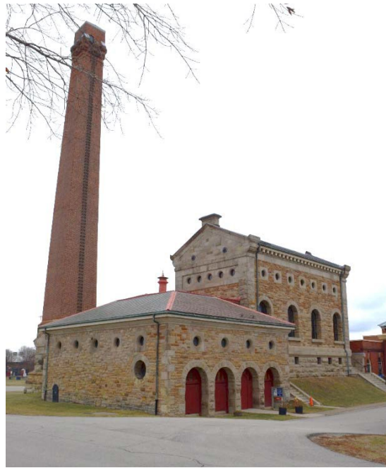
Figure 73: Italianate Boiler House (bottom), and Engine House (top right) of the Hamilton Waterworks (February 2017).
