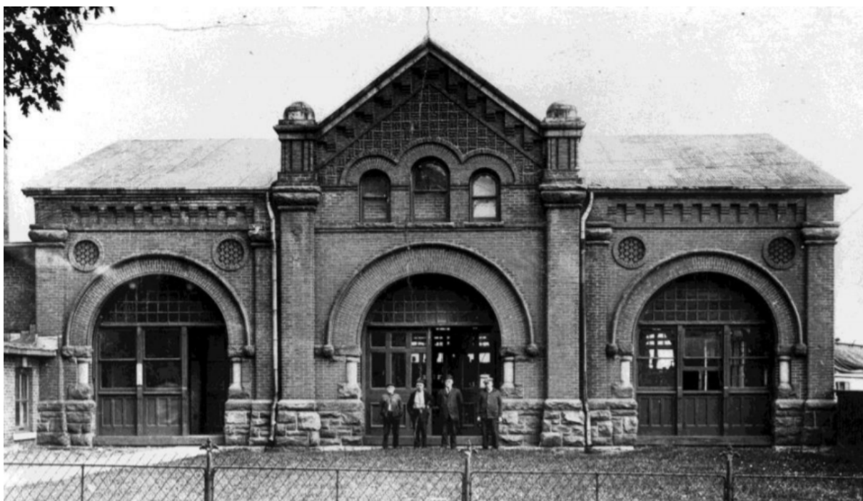
Figure 75: The 1889 Kingston Pumping Station, photographed in 1901 (Wevers 2013:2).
