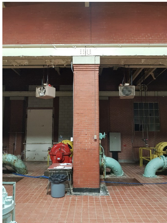
Figure 63: Chamfered and corbelled pillar or column supporting the 1929-30 breach into the 1912-13 Block, as seen facing south from inside the 1912-13 Block.
