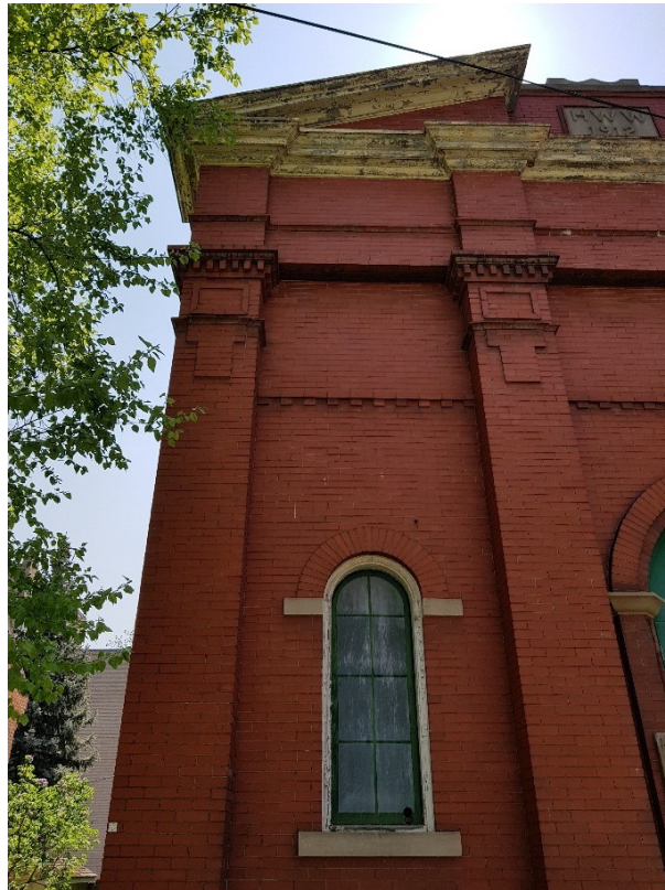
Figure 46: Denticulated string course, pilaster capitals, and entablature above the north bay of the west façade.
