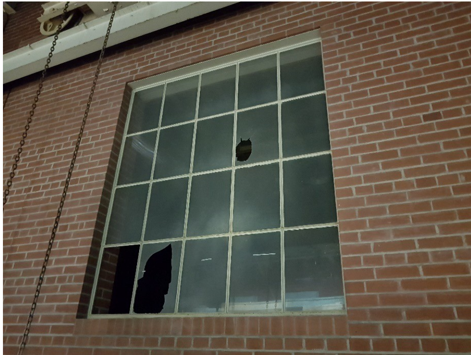
Figure 64: 20-pane fixed sash window on the south wall
