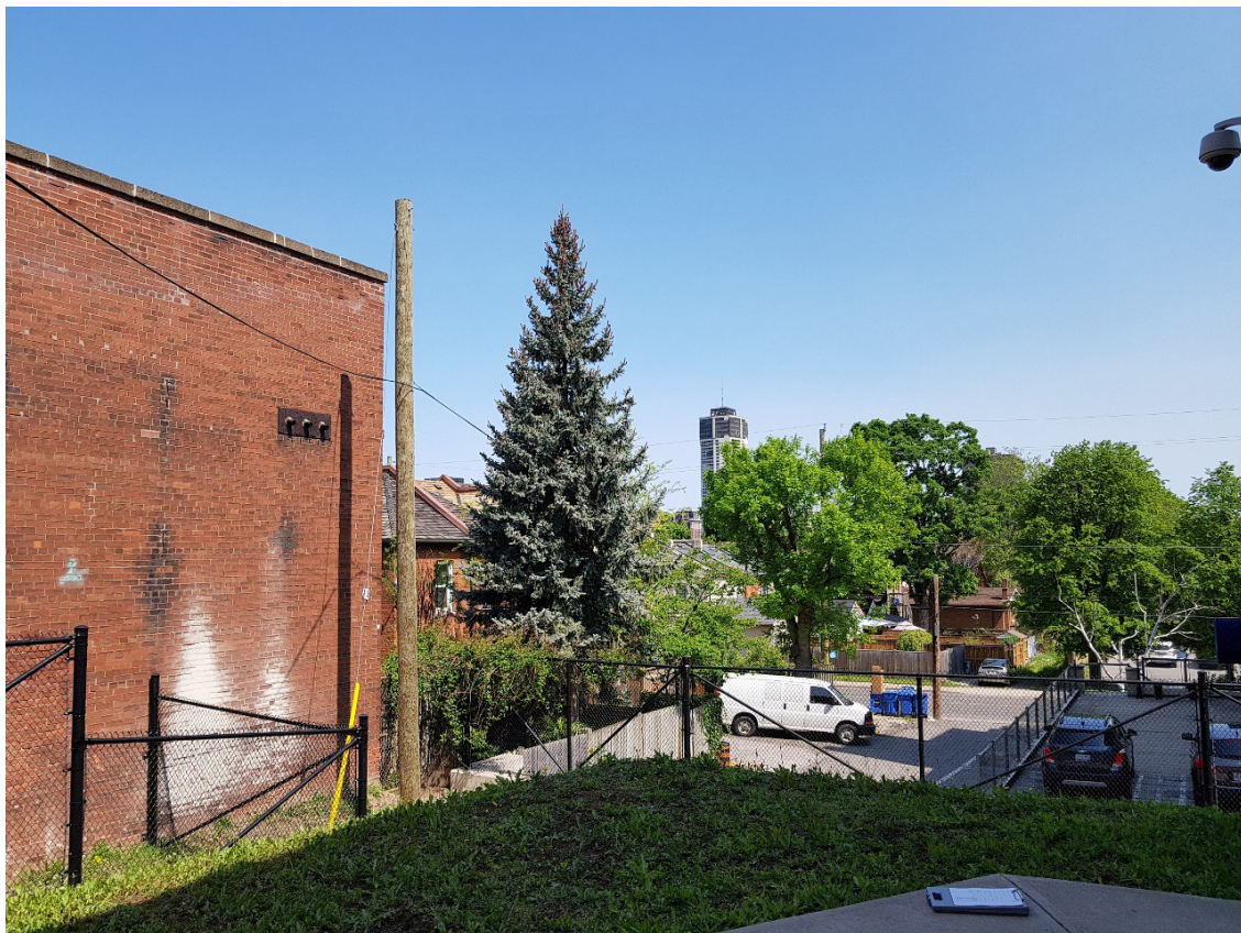
Figure 35: View of the irregular topography and views out from the centre of the property facing northwest from east of the pumping station (far left). The rear sides of the protected heritage properties at 219 to 227 Ferguson Avenue South are visible at centre-left, and the protected heritage properties of 207 to 215 Ferguson Avenue South visible at centre right across Charlton Avenue East.
