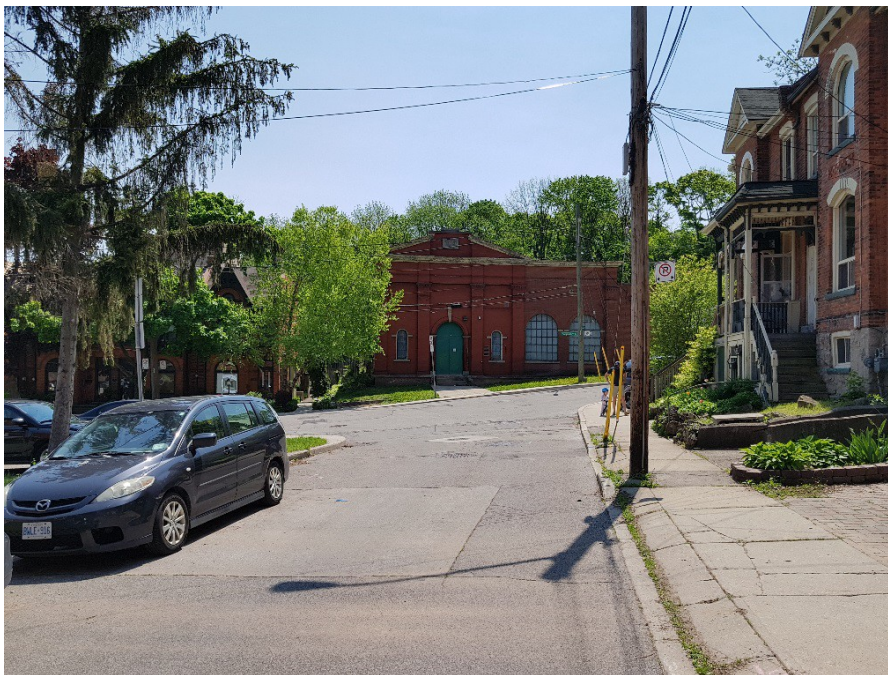
Figure 77: Semi-circular headed openings matching those of the Ferguson Avenue Pumping Station (centre) can be seen on the bottom level of 219-227 Ferguson Avenue (left), and the top level of 32-34 Foster Street (right).
