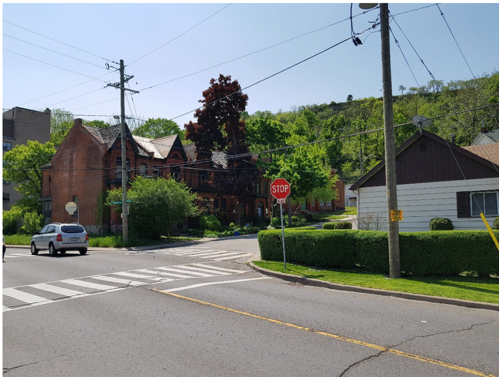
Figure 31: View facing southeast from the intersection with Charlton Avenue East. The pumping station is just visible behind the trees at centre, and the designated heritage properties of 221-227 Ferguson Avenue South are at left.
