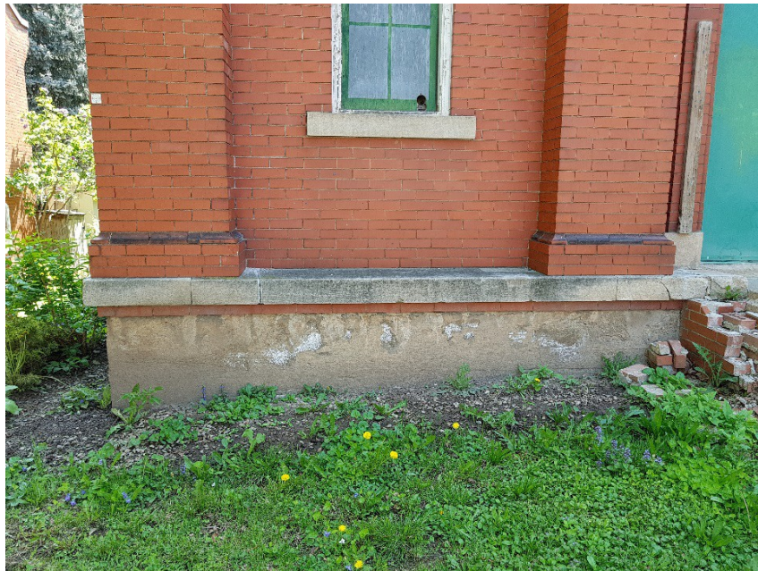
Figure 43: Concrete foundation, pedestal, and pilaster bases at the northwest corner.
