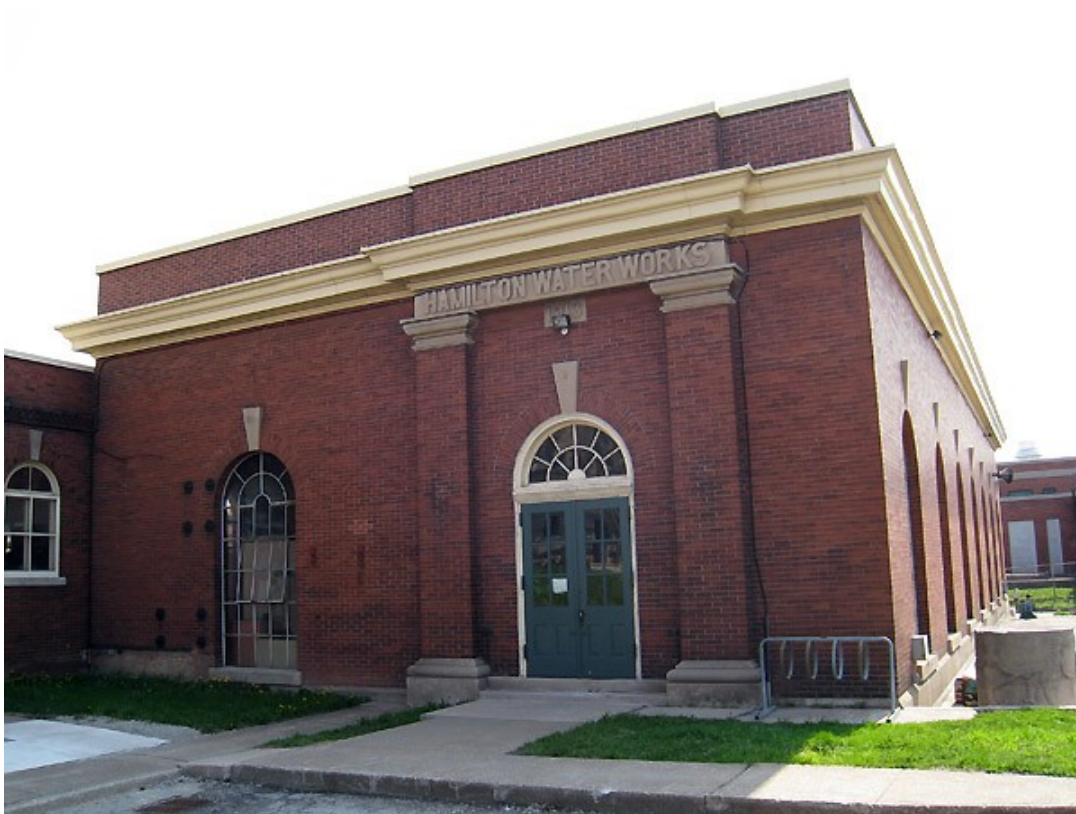
Figure 74: Macallum and Edward's 1913 Pumping Station at 900 Woodward Avenue, designated under By-law 86-310 (photo by Brian Kowalewicz, posted on Historical Hamilton 2009).
