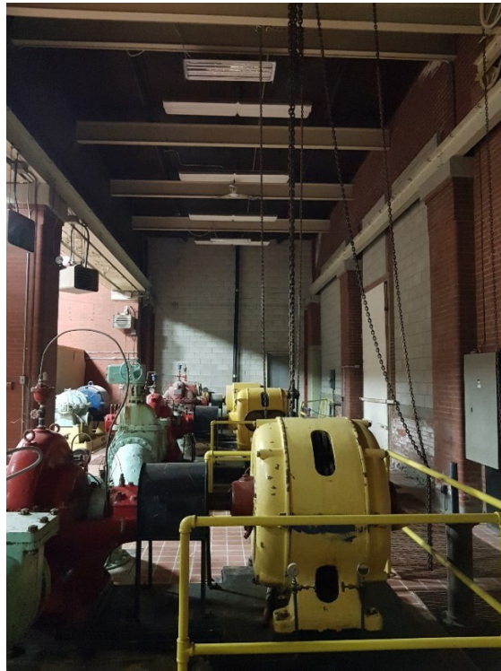
Figure 62: Interior of the 1929-30 Extension, facing east.
