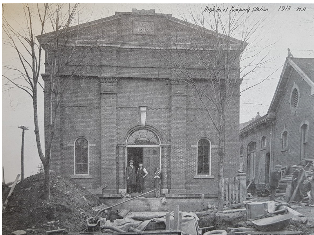
Figure 15: The new pumping station under construction in 1912. The earlier 1878 Repumping Station is visible at right (City of Hamilton 1913).
