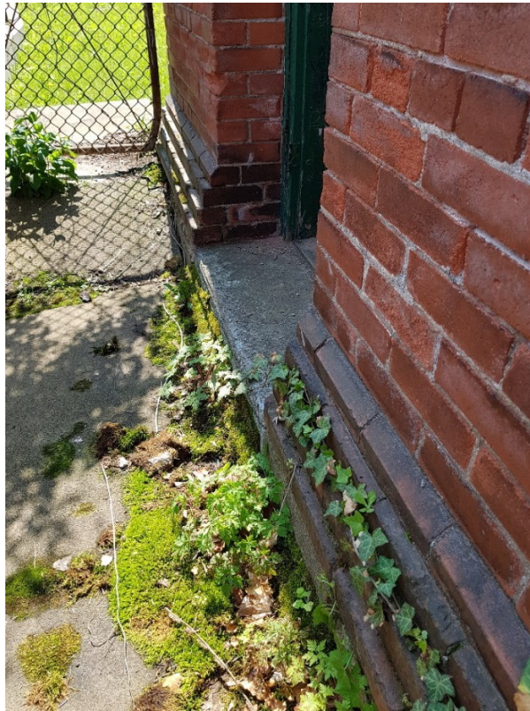
Figure 44: Brick water table at the northeast entrance.
