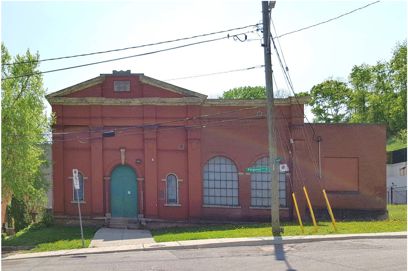
Figure 36: West façade of Ferguson Avenue Pumping Station (rectified to remove distortion).
