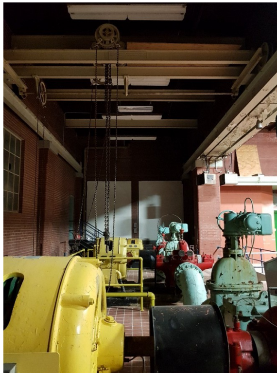
Figure 61: Interior of the 1929-30 Extension, facing west.
