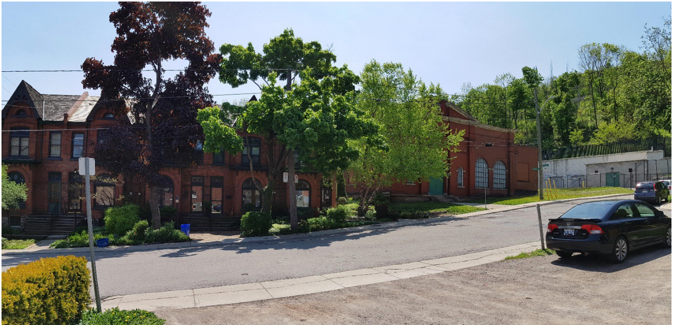
Figure 26: View facing east of the Ferguson Avenue Pumping Station (far right) and protected heritage properties at 219 to 227 Ferguson Avenue South (left).
