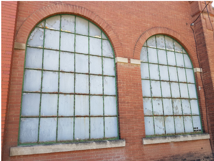
Figure 60: Large windows of the 1929-30 Extension west façade.
