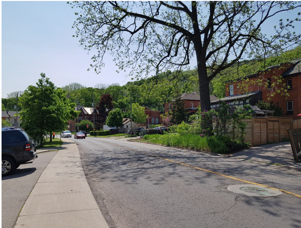
Figure 32: View of the pumping station facing southwest from east on Charlton Avenue East. The 1912-13 and 1929-30 elements of the pumping station are visible at centre.
