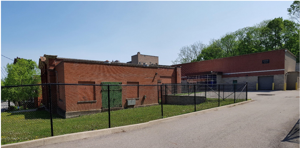
Figure 28: View facing northeast of the Ferguson Avenue Pumping Station (left) and new station (right) showing the irregular topography.
