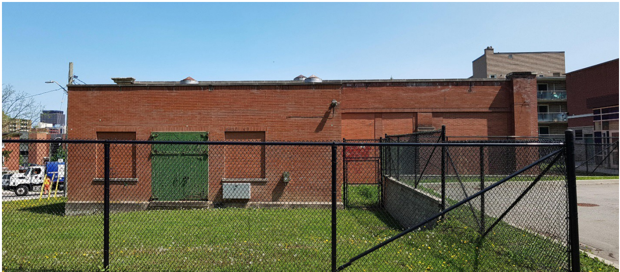
Figure 38: South façade (rectified to minimize distortion).
