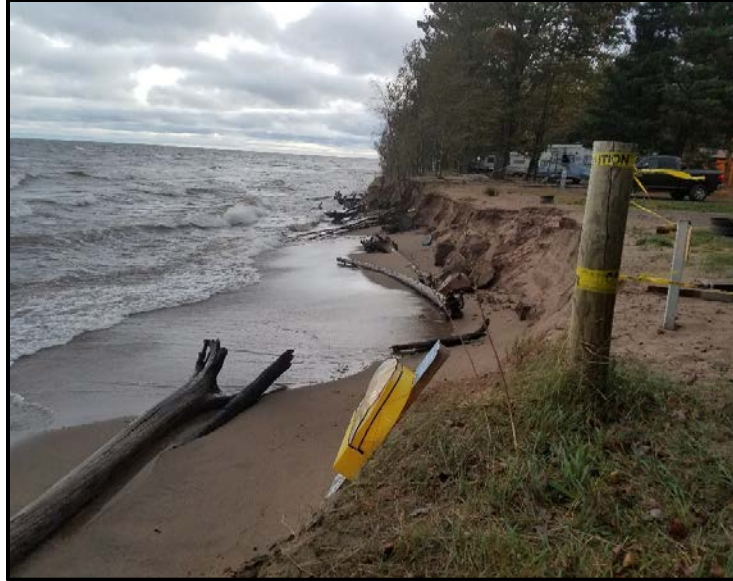
Figure 5-15: Reported coastal erosion at Ontonagon Township Park and Campground. For the past three years staff have been monitoring the rate of erosion and measured 120-ft of shoreline loss since 2014. Erosion has caused closure of selected campsites and impacts to power utilities. Photo credit: Superior Watershed Partnership and Land Trust – Great Lakes Coastal Reporting Tool .
