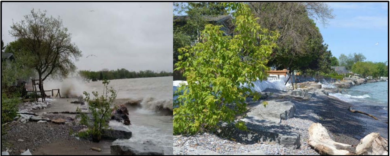
Figure 5-29: Cedar Crest Beach Road. The photo on the left was taken May 25, 2017. Photo credit: Clarington Fire and Emergency Services. The photo on the right was taken June 14, 2017. Photo credit: ECCC.
