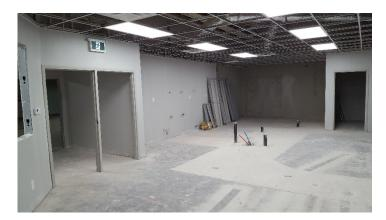
In the photo at right you can see that work in progress. Doors, ceilings etc. are also now completed. The space at the back center is for the walk-in refrigerator and freezer. The door visible back right, will lead to a walk-in pantry. Some of the plumbing and electrical, mid installation is visible in the centre of the picture and on the extreme left you will see the then unfinished pass through opening from the kitchen to the hallway and the rest of the space.
