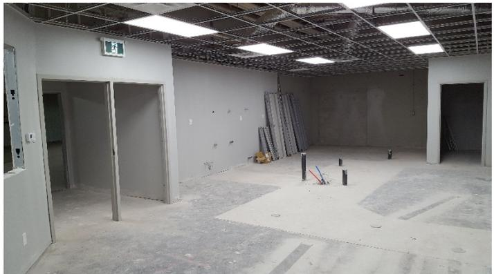
In the photo at right you can see that work in progress. Doors, ceilings etc. are also now completed. The space at the back center is for the walk-in refrigerator and freezer. The door visible back right, will lead to a walk-in pantry. Some of the plumbing and electrical, mid installation is visible in the centre of the picture and on the extreme left you will see the then unfinished pass through opening from the kitchen to the hallway and the rest of the space.
