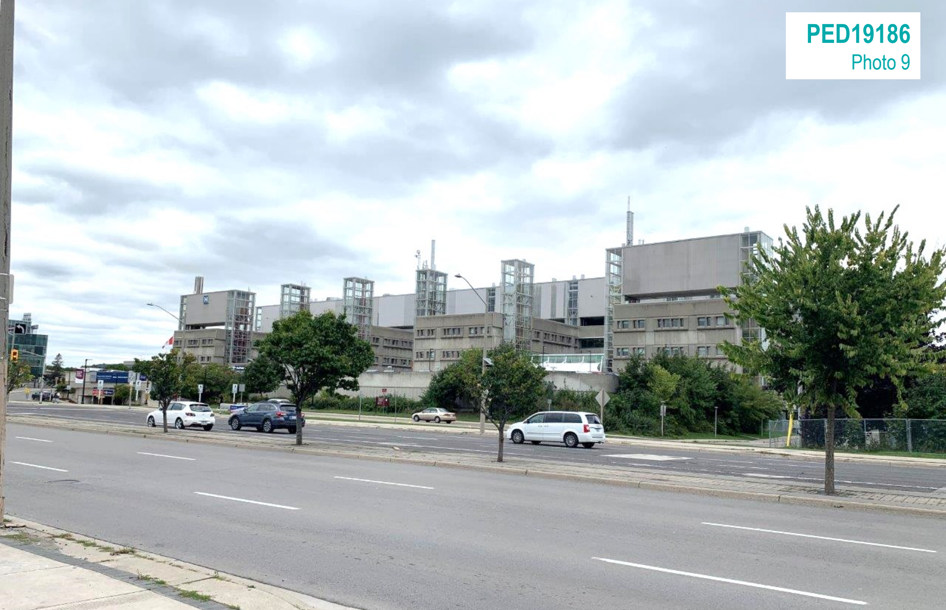
McMaster Hospital to the west
