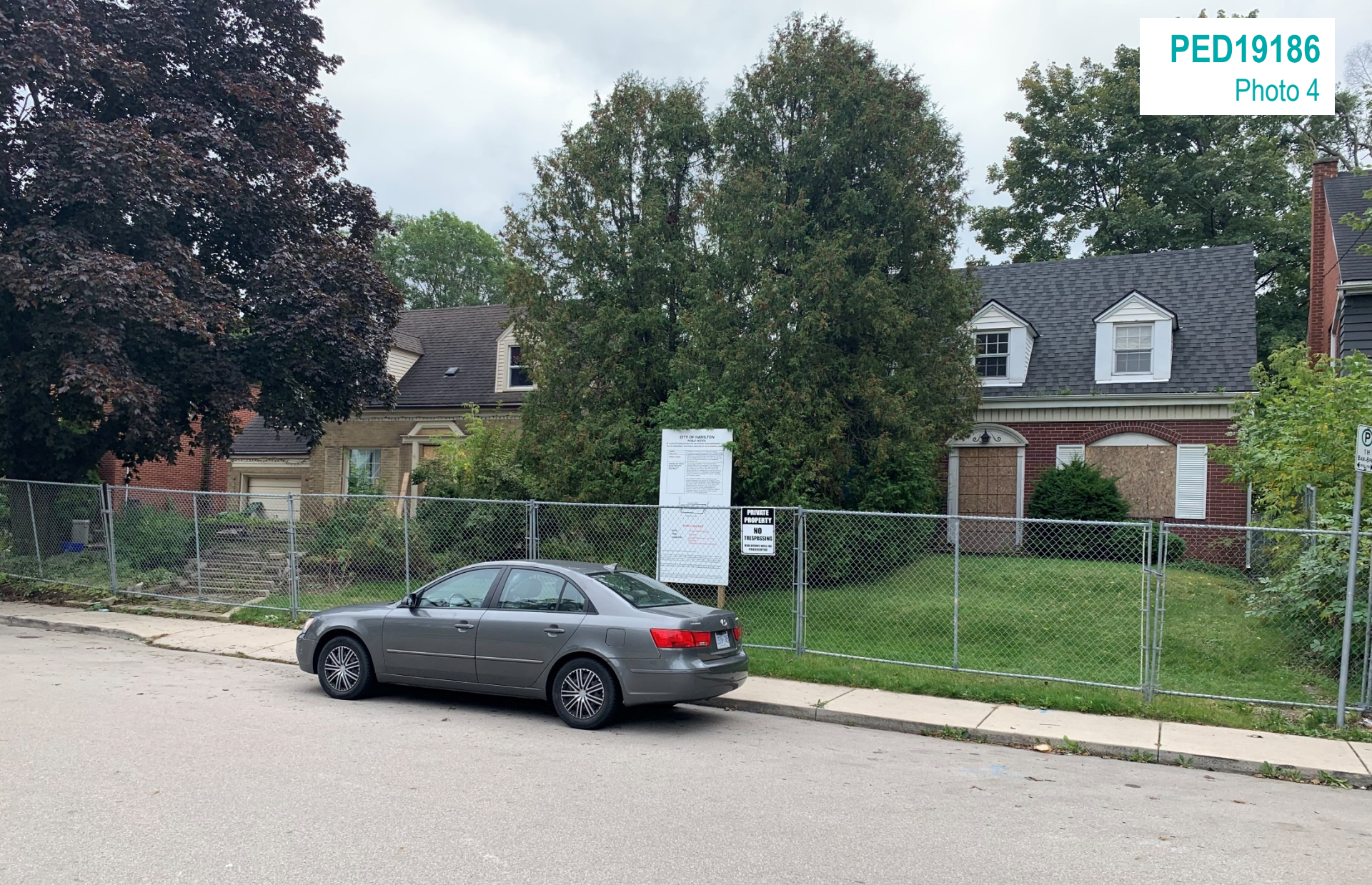
Homes on the southside of Traymore Avenue to be demolished
