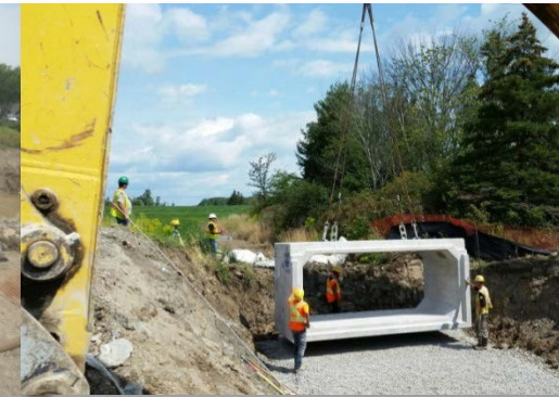
Bell Road Culvert Replacement
