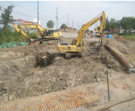
Dartnall Road Culvert
