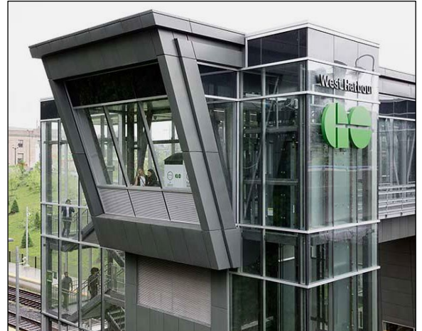
Rush-hour service at West Harbour has doubled through the GO Expansion program
