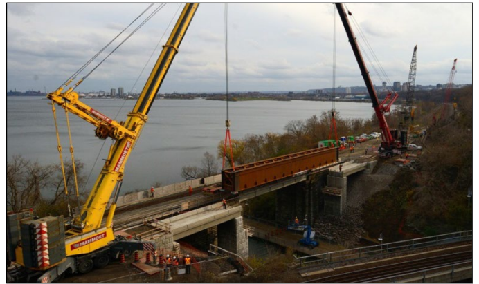
Widening of the Desjardins Canal Bridge
