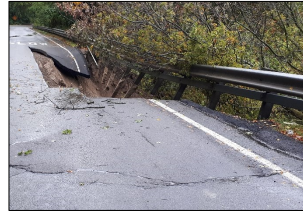
Hwy 8 Dundas Escarpment Failure
