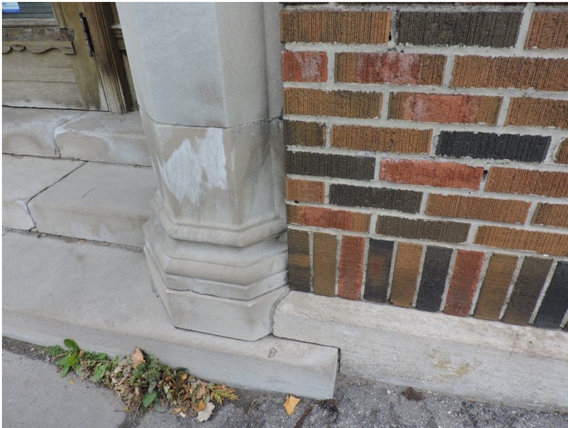
Figure 20 Front entrance, showing concrete steps, pillar base, brickwork, concrete foundation transition (AB, 2018).
