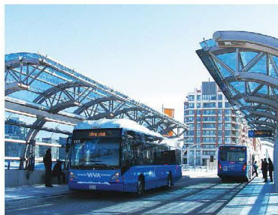
Transportation hubs connect different modes of local and regional transit, are mixed-use nodes, and support higher densities.
