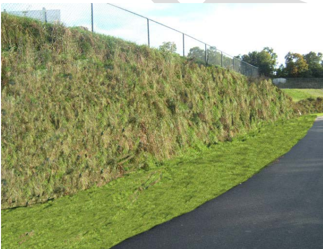
Figure 6.12 Mechanically Stabilized Earth Berm (Strata System)
