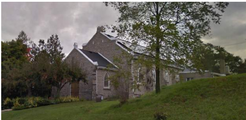
Figure 5.14- West Flamborough Presbyterian Church (source - google maps)
