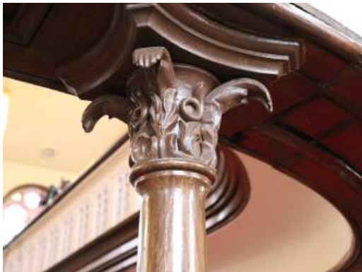
Figure 4.14 - Detail of Column supporting balcony
