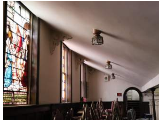
Figure 4.15 - View of ground floor gallery
