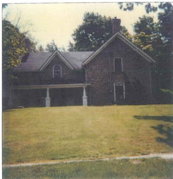
SIDE VIEW OF MILLER'S HOUSE FACING NORTH (WILSON ST.)
