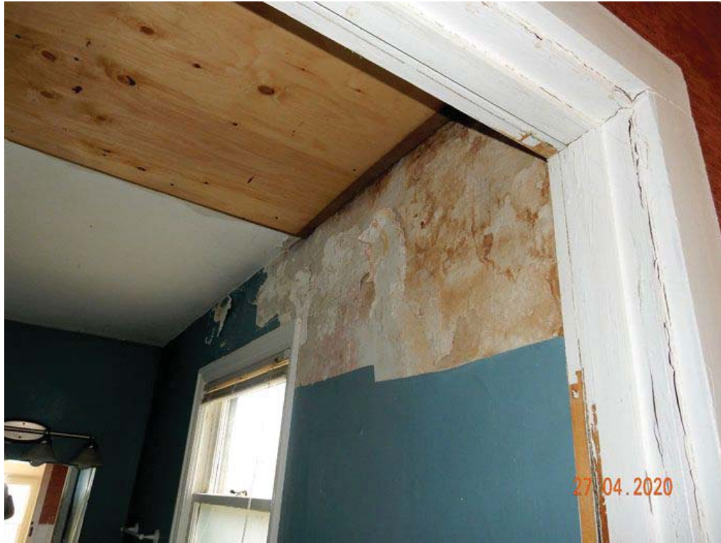
Figure 10: Interior Ground Floor New Trim and Damage Ceiling and Plaster, 1389 Progreston Road
