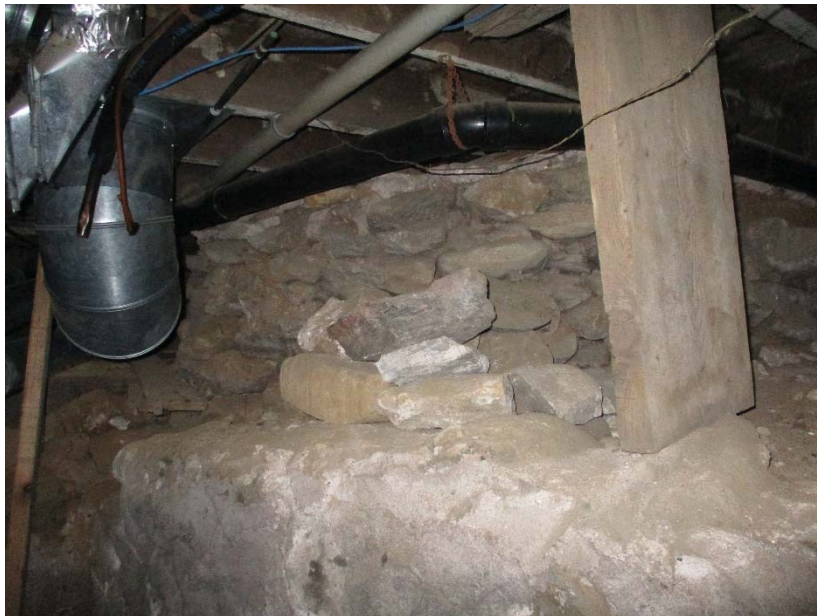
Later basement wall (foreground) supporting earlier shallow wall (background) Also note temporary prop under failing joist
