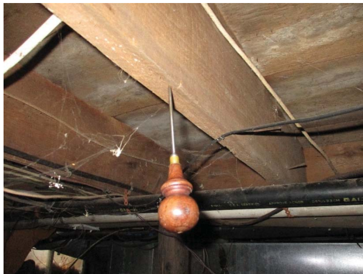
Deteriorated floor joist, awl inserted >2"
