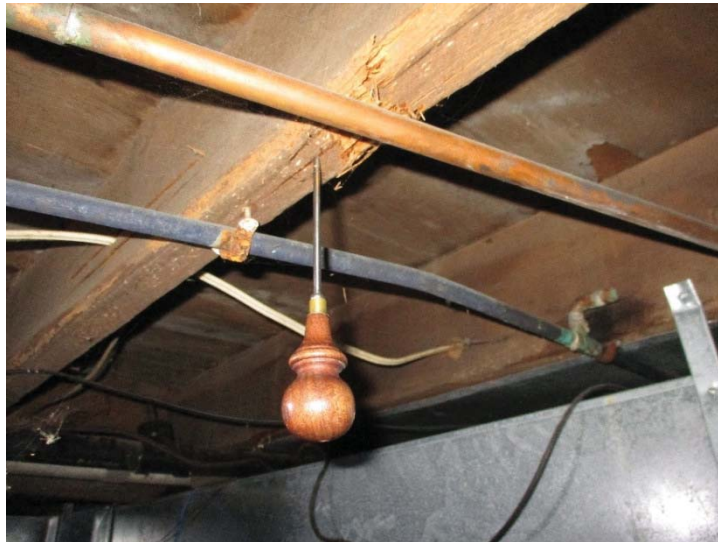
Deteriorated floor joist, awl inserted >2"
