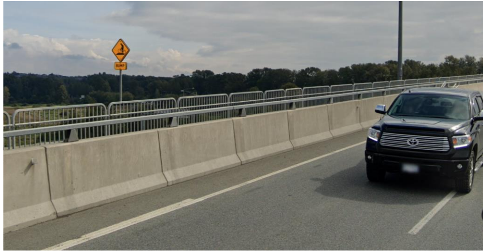
FIGURE 2: BUMP Warning Sign on the Port Mann Bridge 4
