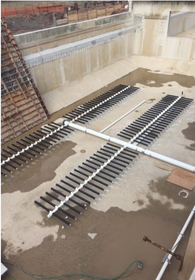
Figure 4: South Aeration Plant Expansion Construction
