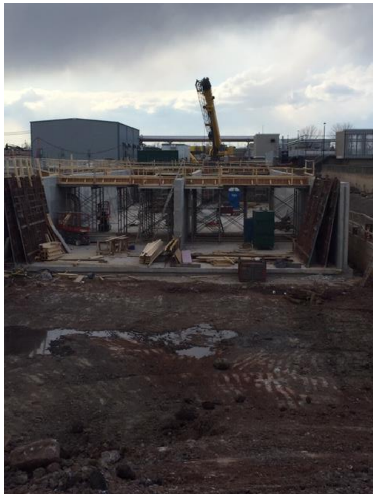
Figure 9: South Aeration Plant Expansion Construction
