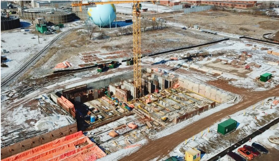
Figure 7: New Tertiary Treatment Facility Construction
