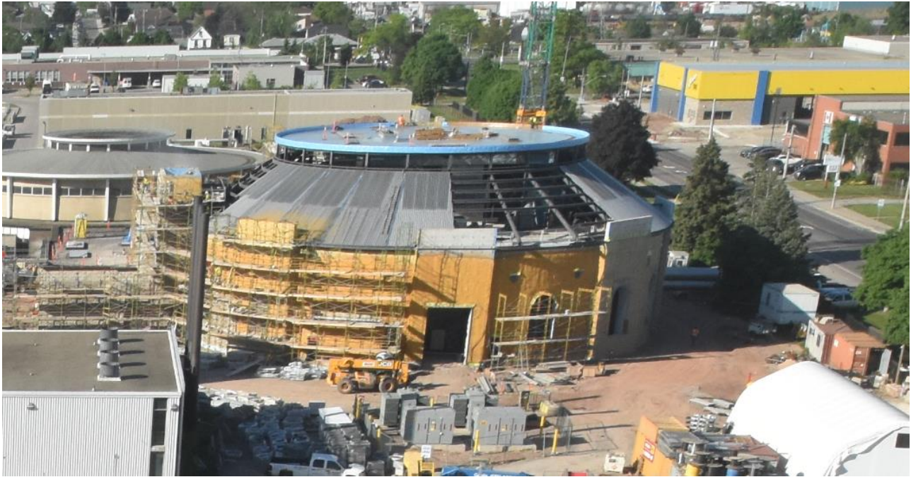
Figure 2: New Main Pumping Station
