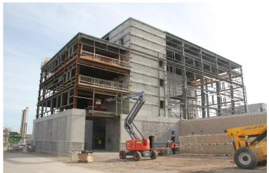
Figure 4: Structural Steel Construction (2019)
