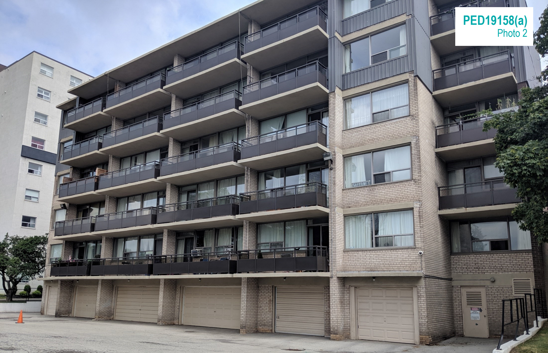
Existing multiple dwelling from the rear
