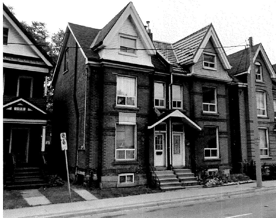
EXISTING BUILDING IMAGE
