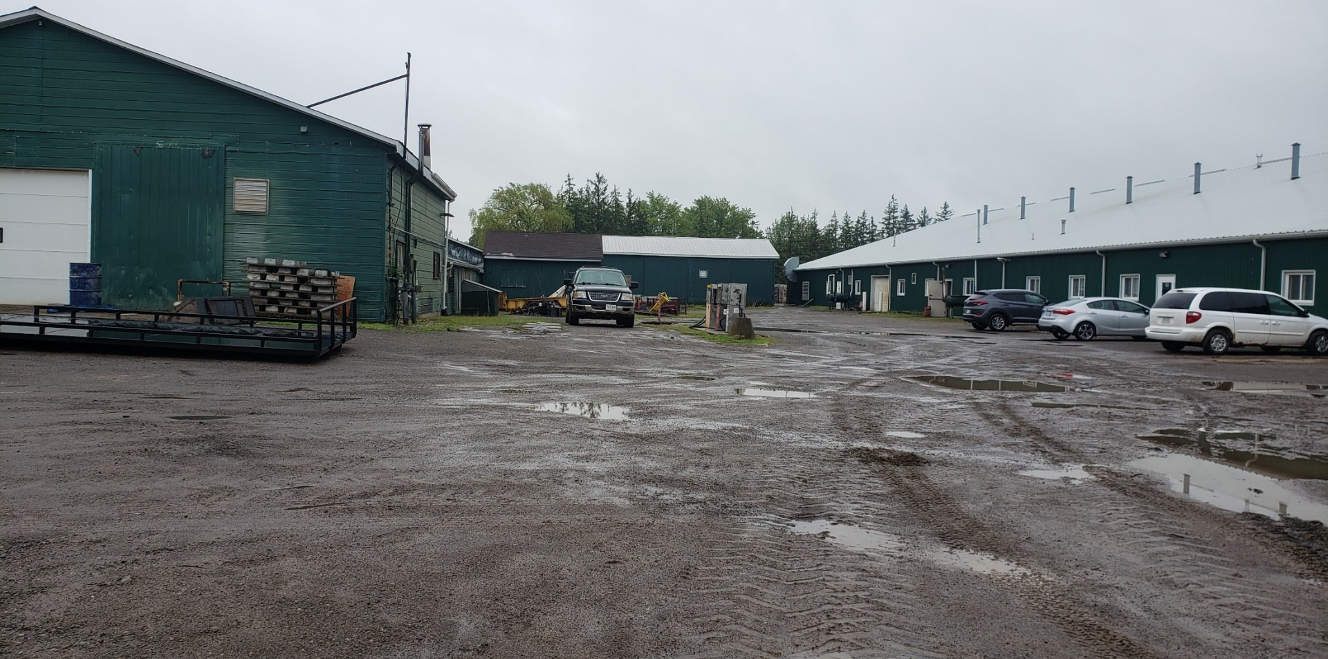
Existing Wire Basket Building
