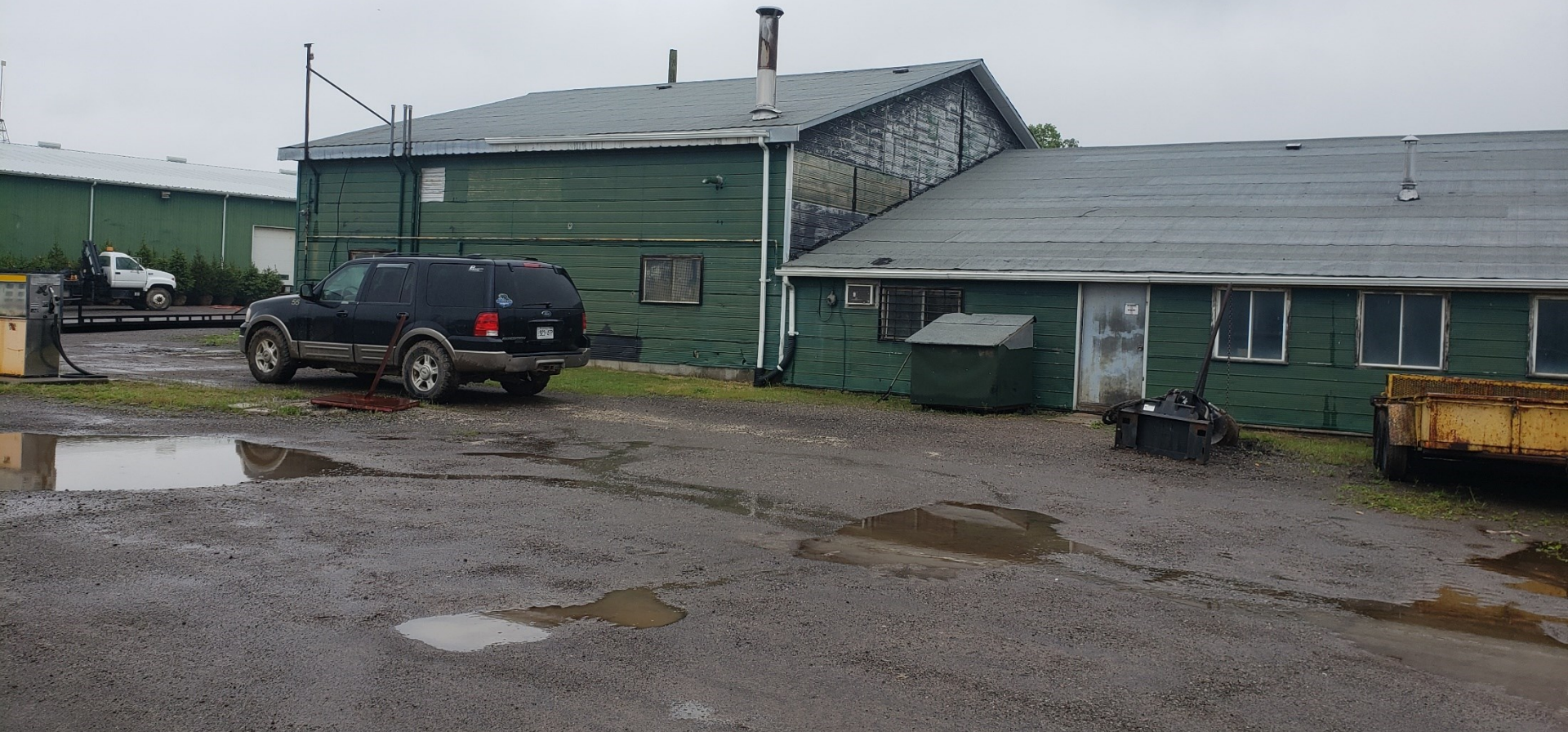
Building to be demolished
