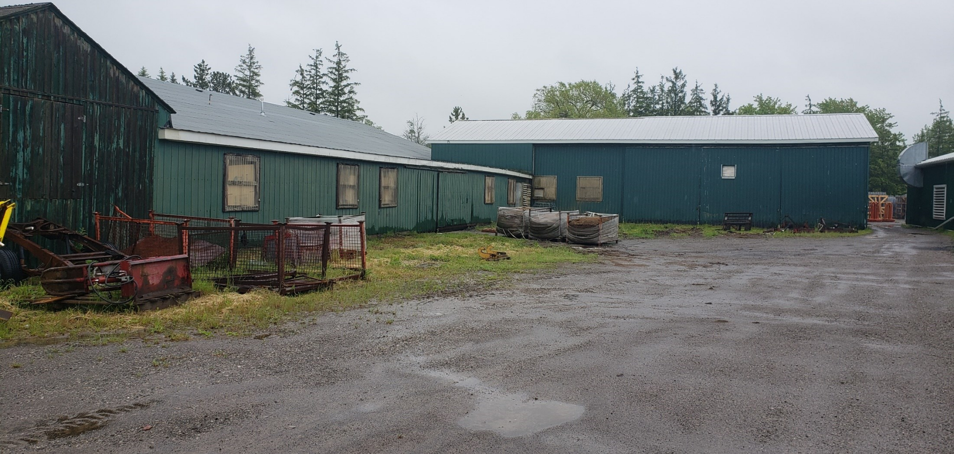
Building to be demolished
