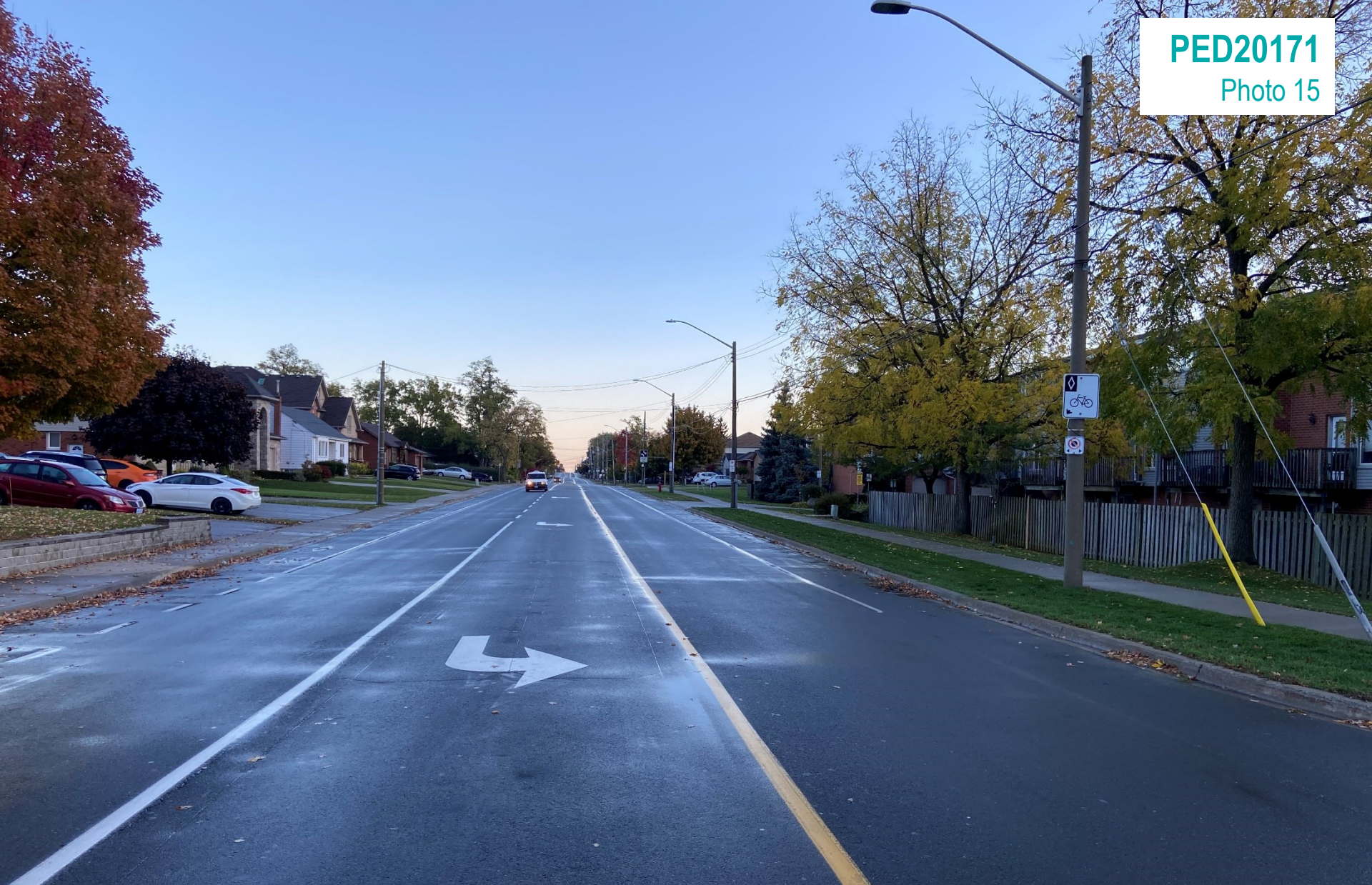
West 5 th Street (looking north)
