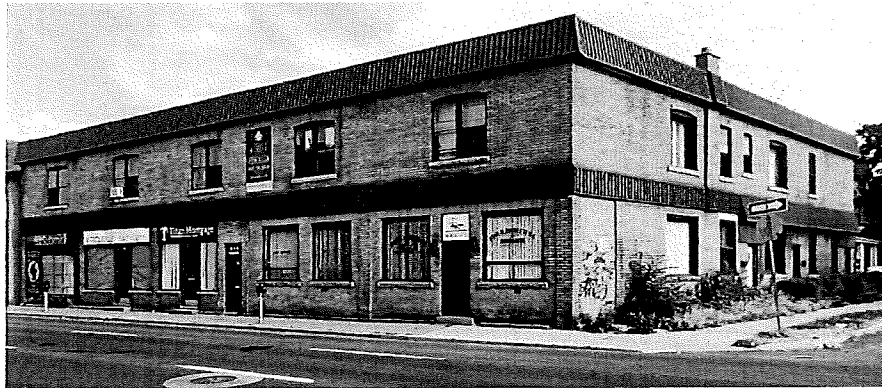
EXISTING BUILDING IMAGE
