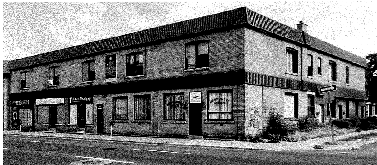
EXISTING BUILDING IMAGE
