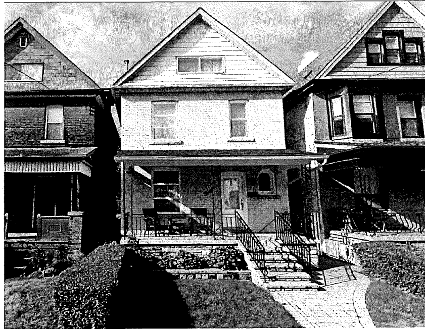
EXISTING BUILDING IMAGE
