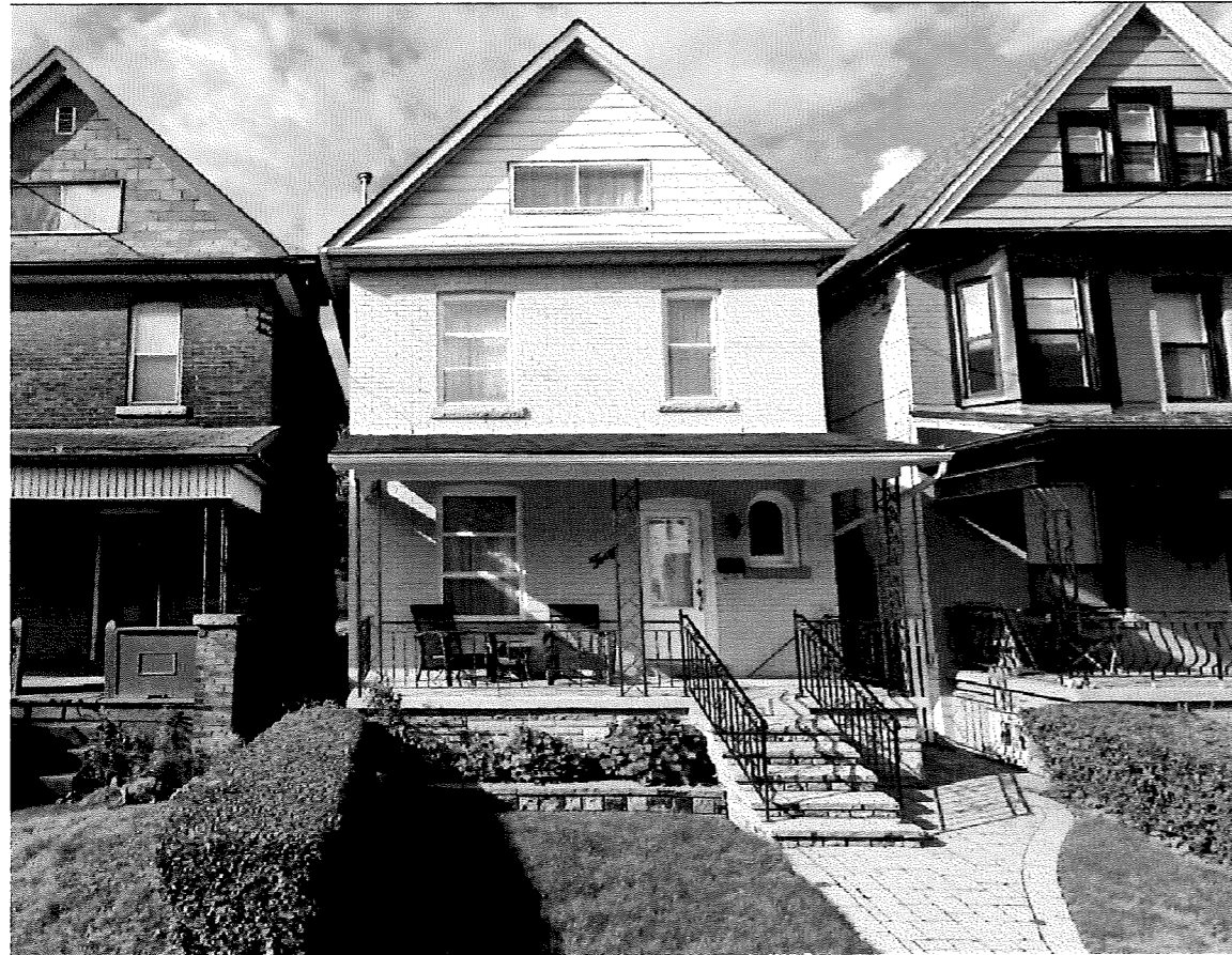
EXISTING BUILDING IMAGE
