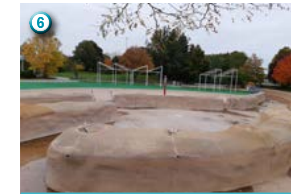
6 Exposed spray nozzle pipe poses a safety risk. Caulked joints are unsightly and collecting mold.
