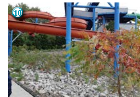
10 Loose rocks under the east slides work pose a safety hazard.
