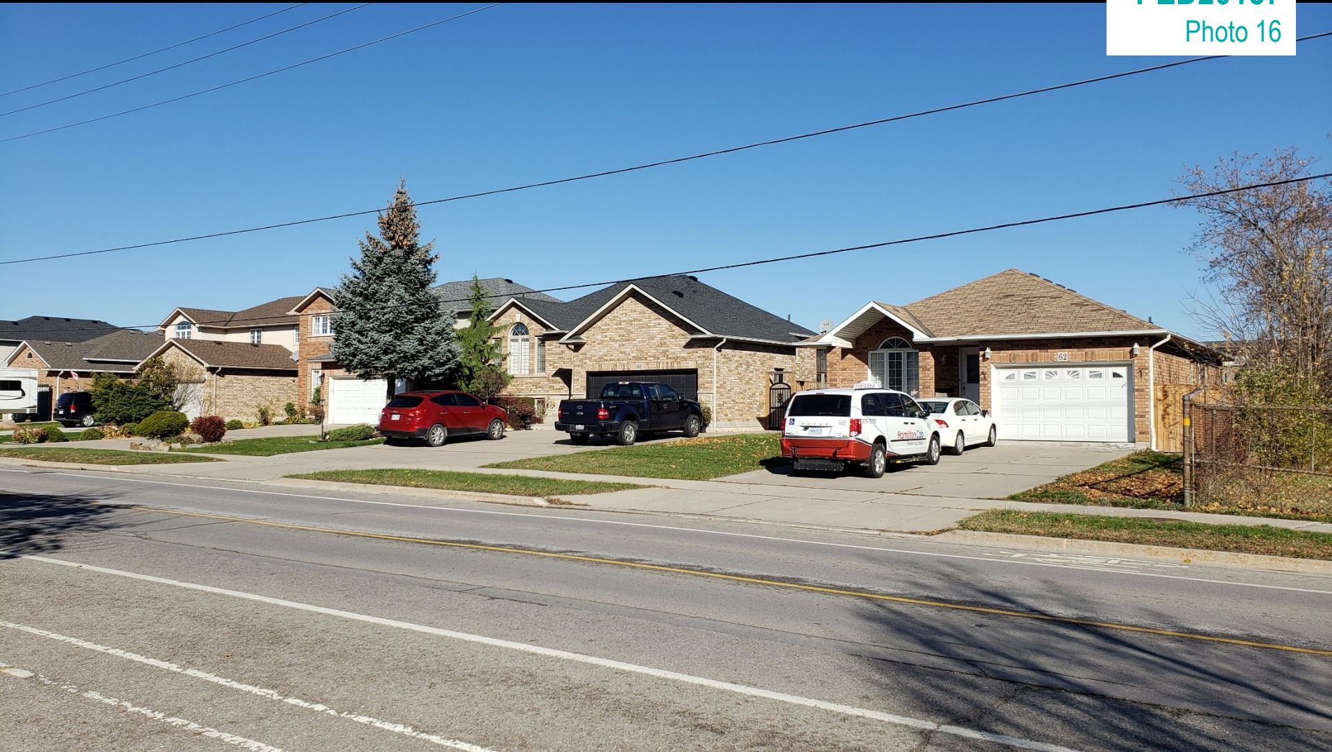
Single detached dwellings along Highland Road West to the west
