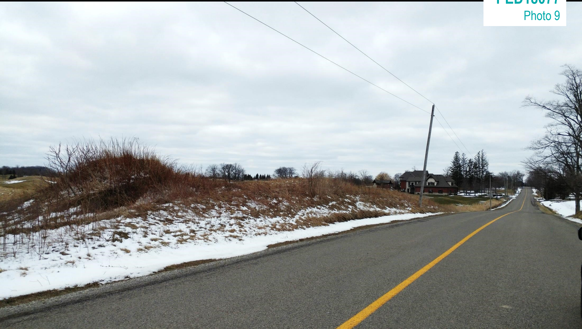
Looking east of the Subject Lands along English Church Road East
