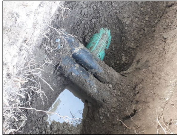
Sewer lateral damage – Markland St.
