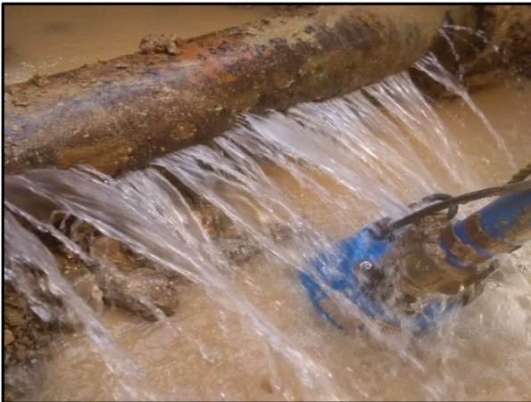
Watermain break – Waterdown (Dundas St.)
